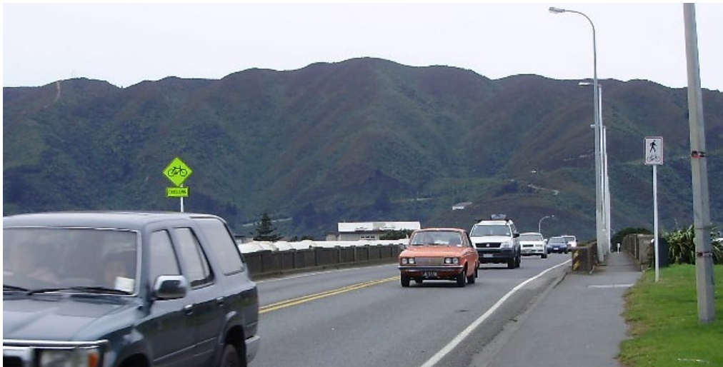
Figure 19 Pedestrian Facilities on Waione Bridge
