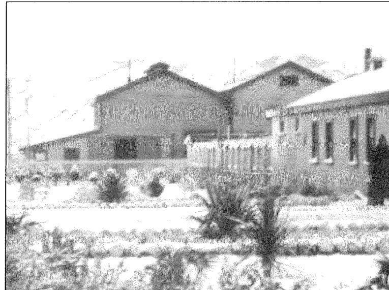
Featherston Camp Building prior to demolition. ATL 08-061-004a.
