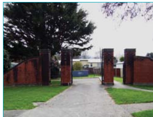
Tidy up and brighten the gates and entrance from Tocker Street
