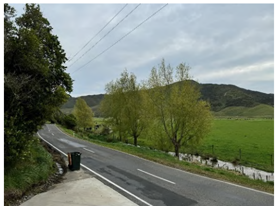
Figure 8 - Typical view of northern fill zone from Coast Road 12/09/2024
