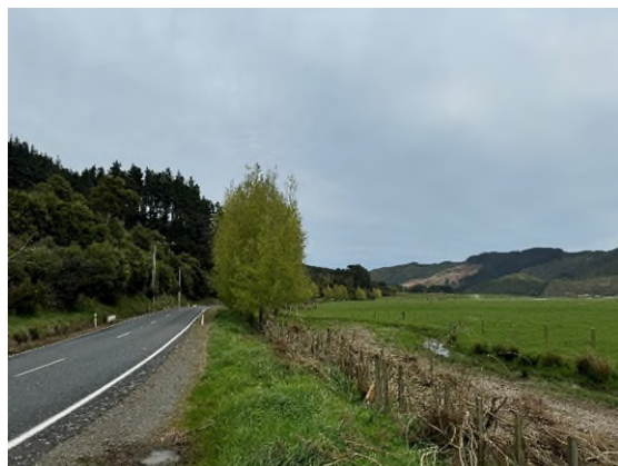
Figure 7 - Typical view of northern fill zone from Coast Road 12/09/2024
