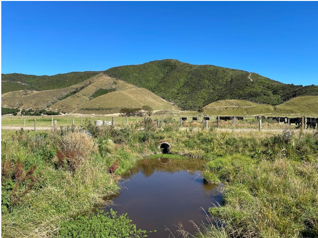
Figure 6: Photo 4. Culvert crossing where the existing farm access track crosses the northern intermittent stream. Photo taken on 22 January 2025.
