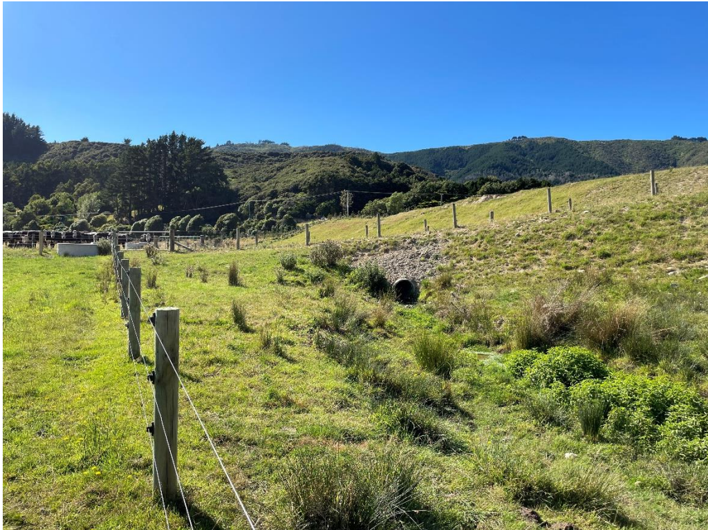
Figure 7: Photo 5. Culvert crossing where the existing farm access track crosses the northern intermittent stream. Photo taken on 22 January 2025.
