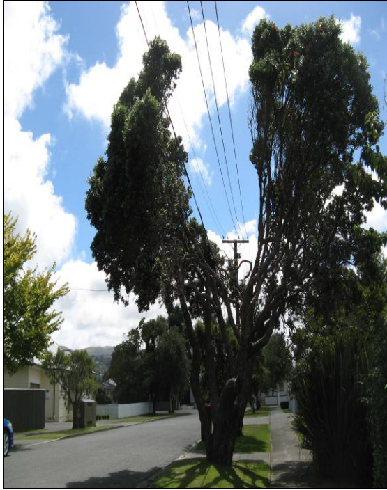
Local V pruning of pohutukawa to accommodate 400V lines
