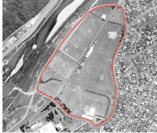
Figure 13 - 1988, the park is again extended after the adjoining Webb's Shingle Works is closed, cleared and grassed over
