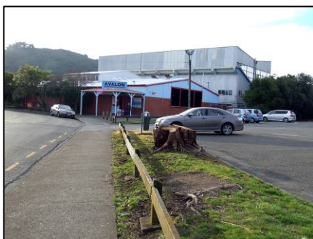
Figure 36 - Avalon Rugby Football Club with bar and TAB facilities
