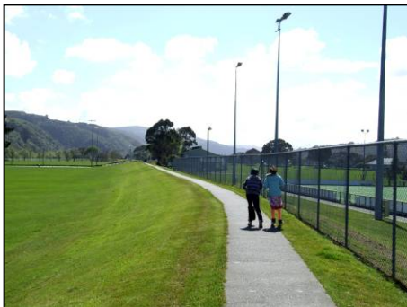
Figure 25 - Concrete pathway along the top of the stopbank
