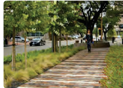
Figure 14: Bagby Street Reconstruction, Houston, Texas
