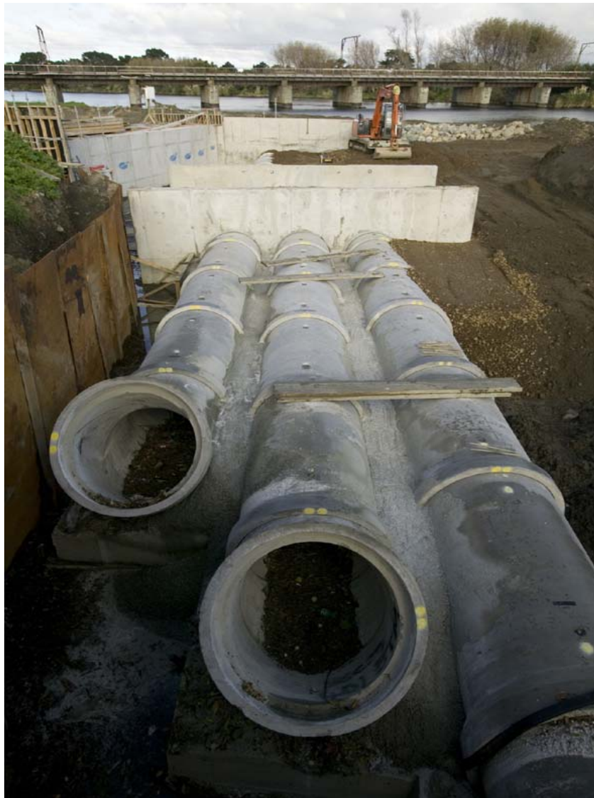
Construction of the Oahu Stormwater Pump Station (2006)
