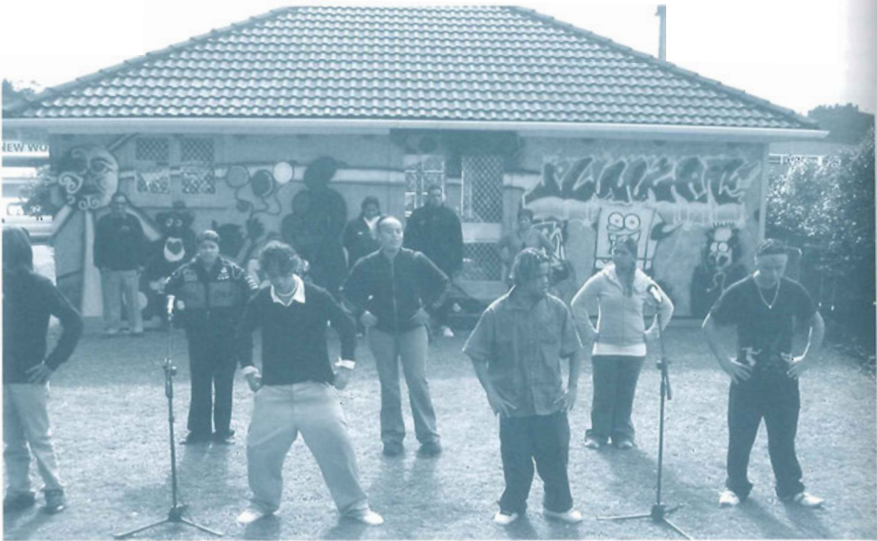
A team of students from Korauui Marae was involved with Cr. Angus Finlayson in the repair of the Plunket Room exterior walls. A second team was involved with Council's contracted artist to create the child friendly murals on the walls facing the children's playground in Speldhurst Park. The story of this project has been captured in a children's storybook which is read to pre-schoolers in the city's community libraries.
