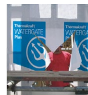
On arrival of doors and windows, cut Watergate at each opening on a 45° angle away from each corner. Pull the Watergate flaps inside and fasten to the inside of frame.
