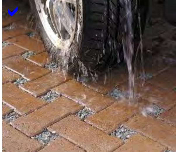
It is important to minimise impervious surfaces by using porous paving as much as possible to reduce to stormwater run off
