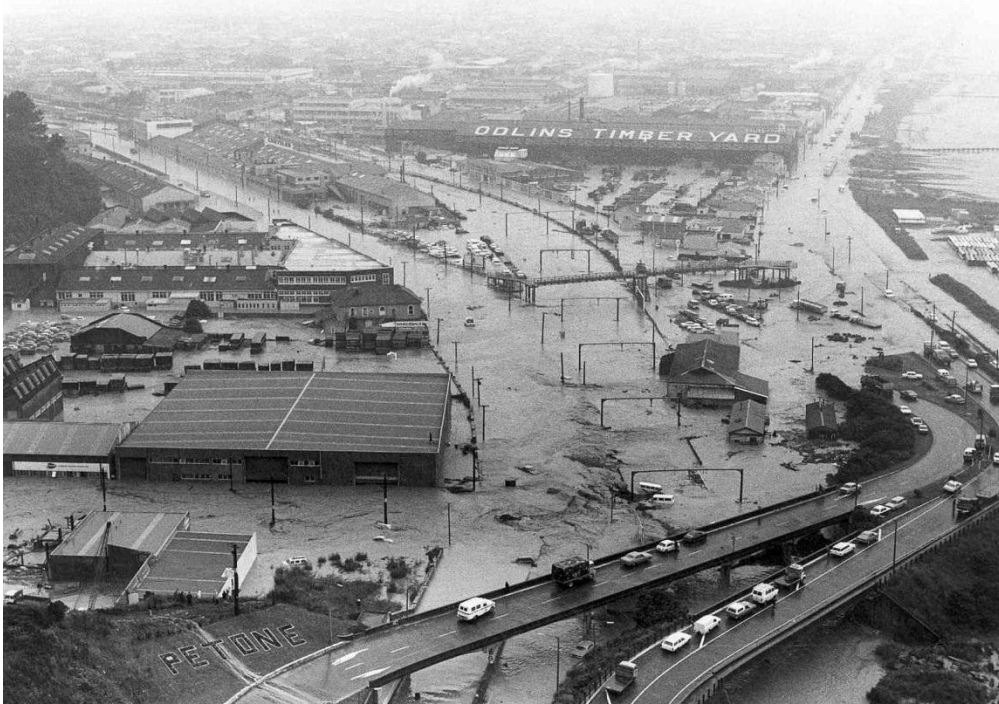
Figure 1 – Flooding December 1976 at Odlins Timber Yard, Petone
