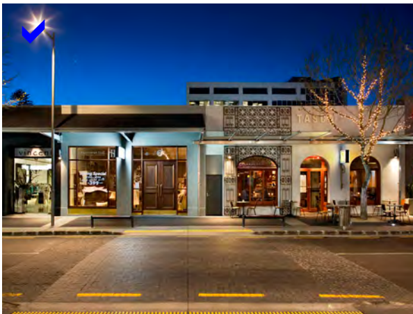
Long frontage modulated at intervals of less than 10m by change in uses (various shops and restaurants) materials, colours, good use of sheltering elements, high percentage of transparent glazing and public/private lighting
