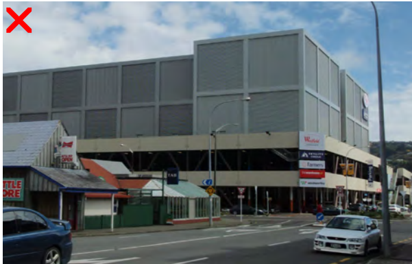
Car parking structure dominates the streetscape; inactive street edge and elongated blank walls
