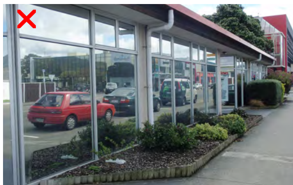
Reflective windows do not offer visual connection between interior and exterior - "cannot see through".
