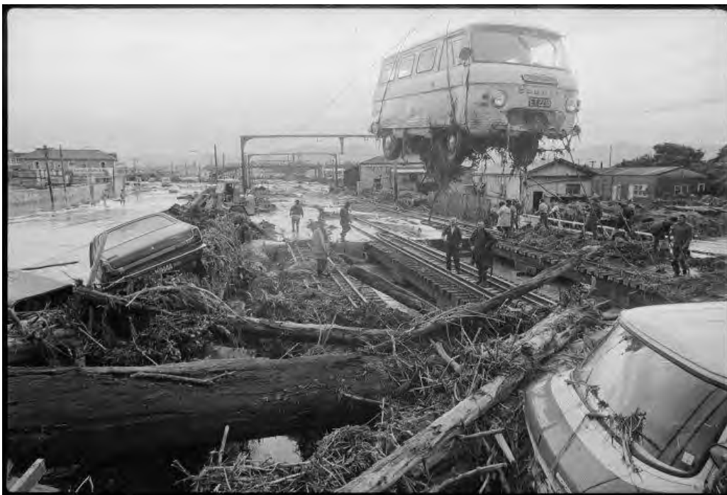
Figure 2 – Flooding December 1976 – Debris removal at railway overbridge, Petone
