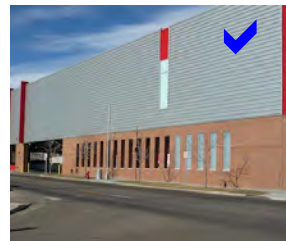
This building has its horizontal length broken up with slot like openings and a material change mid height by the vertical or projecting sections at regular spacings.
