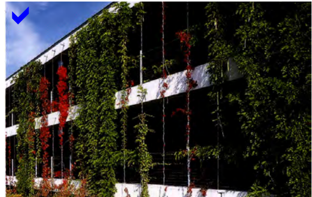
Green walls are a good solution to minimise negative visual impact of car parking structures
