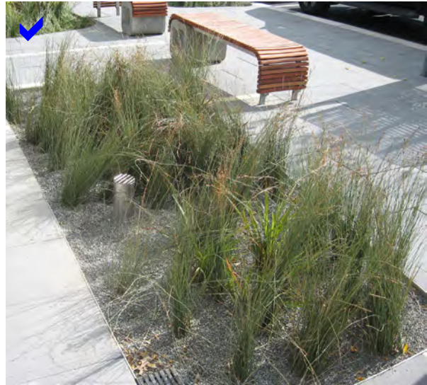
Stormwater devices can be incorporated into the landscape design of new developments.
