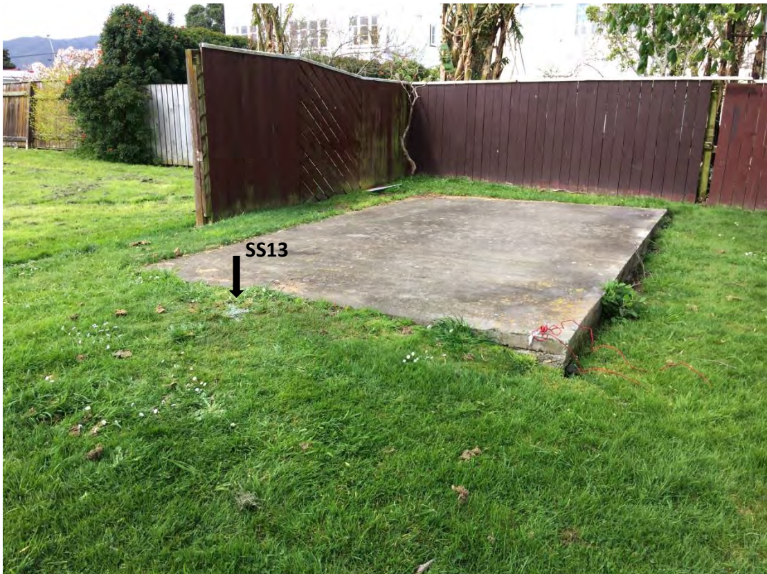
Photograph 6: Northeast corner of the site, looking southeast. The photograph shows the foundation of a shed and sampling location SS13.
