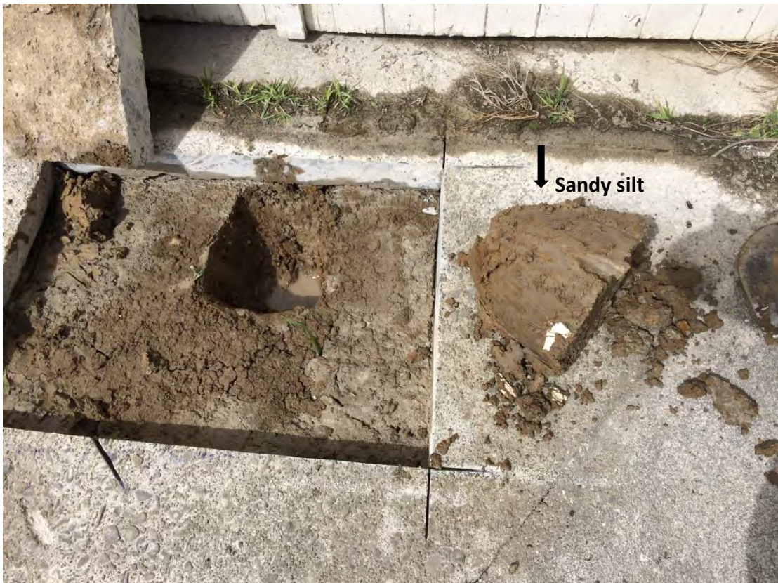
Photograph 8: View of SS11 showing the concrete cut area.
