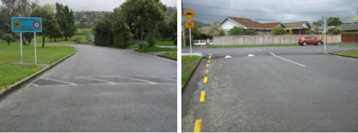
Photos 1 & 2: Access Road to Avalon Park
