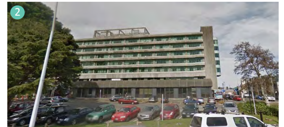
Fig 2.1.22 Hutt Hospital 6-7 stories
