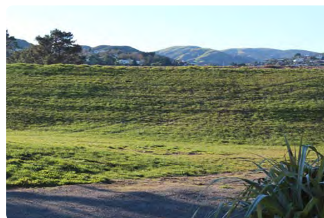
Fig 5.1.3 Rise of the new stopbank on the northern edge of the DPC site Boundary.
