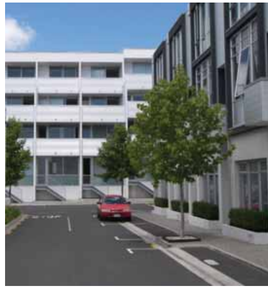
These buildings have floor levels expressed vertically with recessed balconies/windows and the buildings' long horizontal length is visually broken up by the vertical sections at regular spacings.
