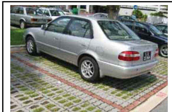
The use of a semi-porous surface allows for stormwater to penetrate through to the ground beneath and also provides some 'greenness' to the area.
