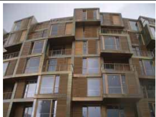
This building expresses each floor level and has recessed and projecting architectural elements as well as different textures to reduce bulk.
