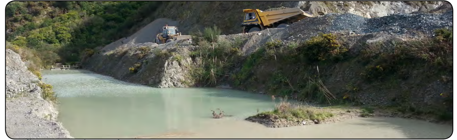
Sediment Retention Pond
