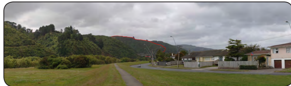
Viewpoint 5 taken from Hutt River Stop Bank adjoining Harcourt Werry Drive looking north
