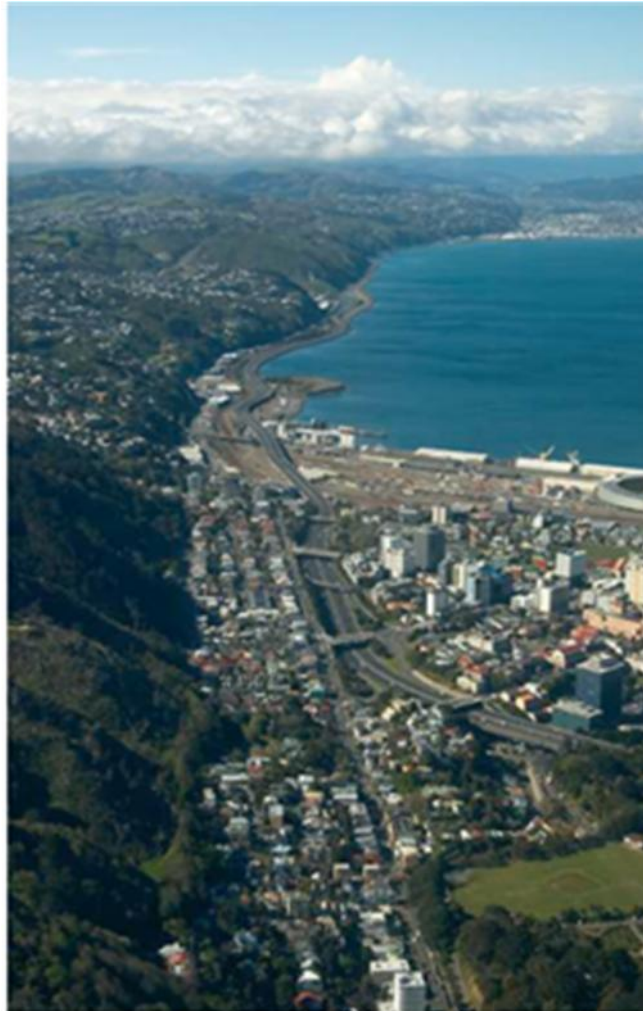
Figure 3. Wellington Fault, looking northeast
