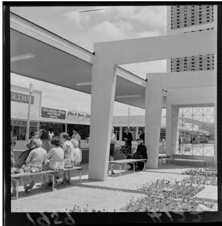
Exterior courtyard showing veranda and cantilevered beams. (Source: EP/1959/3518-F)
