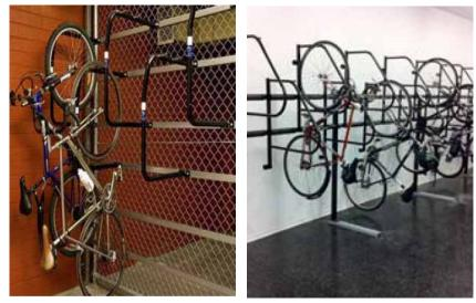
A mix of vertical and traditional stands can both maximise the space that is available and ensure cycle parking is accessible for all cyclists.
