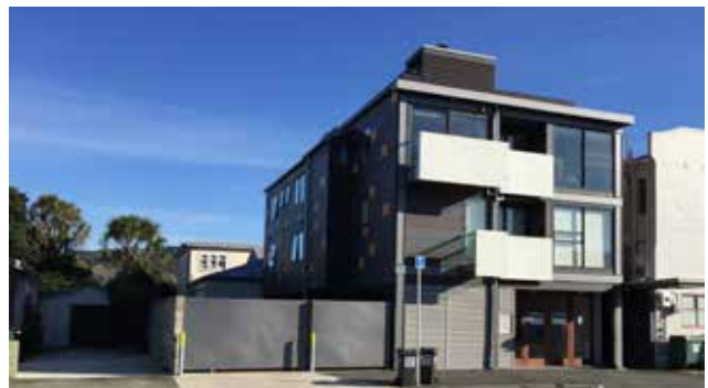
The photo above shows how building placement has reduced potential effects on the adjoining residential dwelling by positioning garaging and access to the side, providing a buffer with the adjoining residential property. The building design also includes modulation, windows and material variation.
