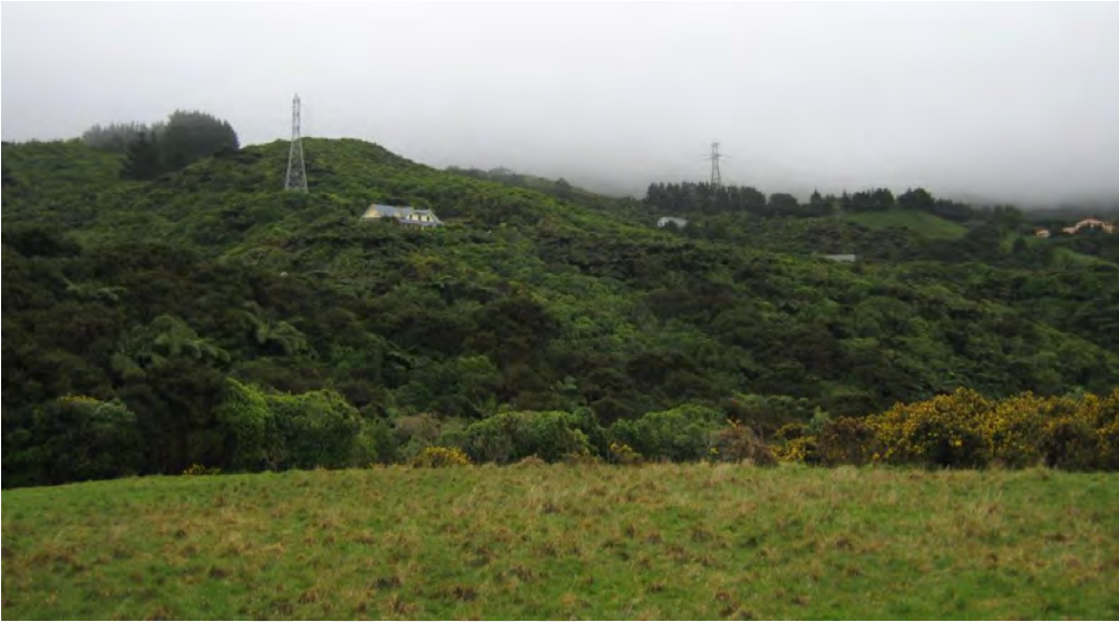
View, nearly due north, across LH009.00 Kaitangata Crescent scrub from 280 Major Drive, Kelson.
