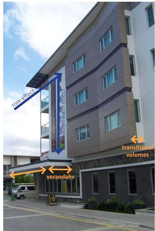
Verandah and transitional volume minimise the adverse effect of increased wind flow
