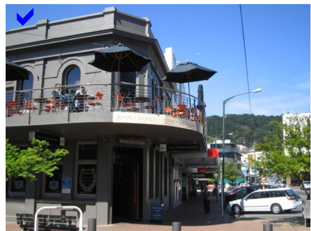
Building faces both primary and secondary street, provides shelter (balcony cover) and visual connection (large proportion of transparent windows on the ground floor with balcony and windows above)
