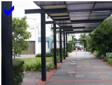
Covered walkways that allow for planting to grow up and over the structure
