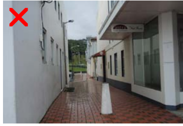
Pedestrian lane gives the impression to be an unsafe environment. Inactive frontages, low levels of transparency, poor attention to details such as signage, landscaping and lighting.
