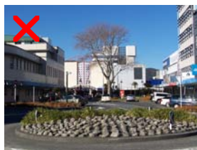
Current building on prominent site
