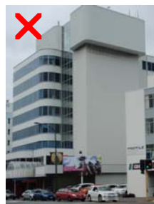
Taller building - blank side wall
