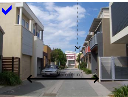
Rear lanes in medium density residential developments. "Eyes on the lane" - studios above garage with balconies and windows facing the lane. Landscaping, lighting and screened bins also enhance its appearance
