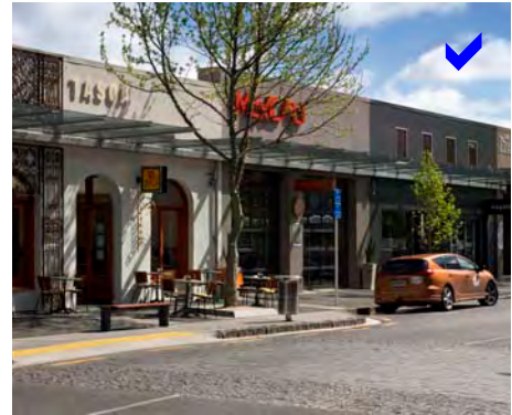
Shops and cafes fronting the street, transparent windows, active use of the sidewalk, residential above retail with balconies facing the public realm
