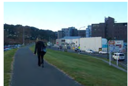
Riverfront (Core) existing character - inactive frontages to the riverfront reserve ("back of the buildings") and vertical separation; a place for "cars and convenience"
