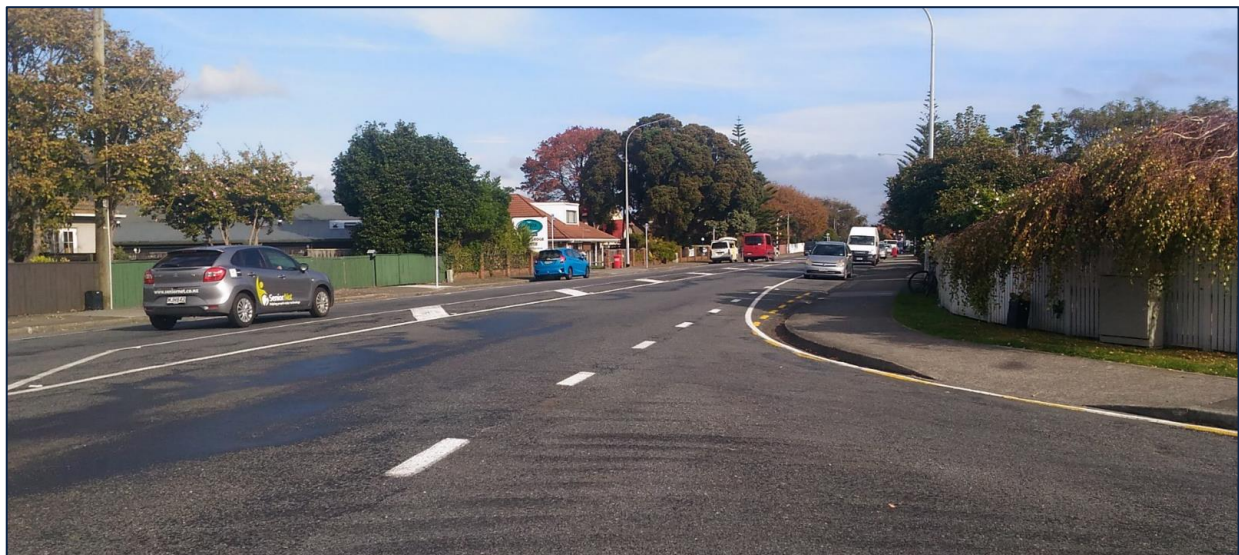
Figure 15 Driver View Exiting Kingston Street – Looking South
