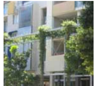
Green structure as part of the facade
