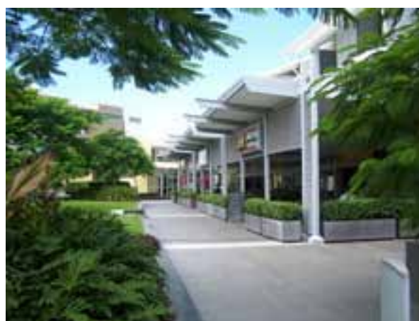
Restaurants fronting onto the promenade and the park, continuous verandahs, high quality landscaping, vertical screens for shade in summer; appropriate signage and quality materials
