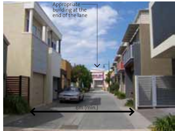
Rear lanes in medium density residential developments. “Eyes on the lane” - studios above garage with balconies and windows facing the lane. Landscaping, lighting and screened bins also enhance its appearance
