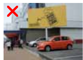
Signage not related to the building
