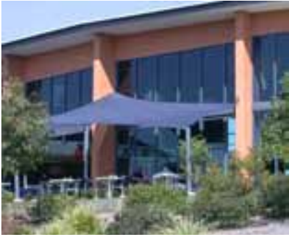
Commercial building that incorporates landscaped buffer and transparent windows facing the courtyard. Facade treatment at small intervals to minimize the bulky appearance
