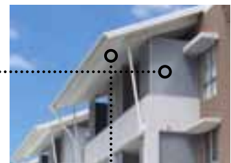
Eaves and moveable vertical shading device (external venetian blind) on east or west facing windows
