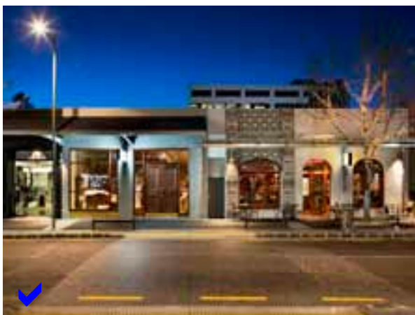
Long frontage modulated at intervals of less than 10m by change in uses (various shops and restaurants) materials, colours, good use of sheltering elements, high percentage of transparent glazing and public/private lighting
