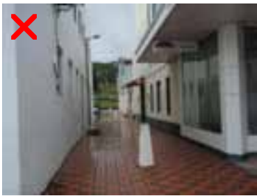
Pedestrian lane gives the impression to be an unsafe environment. Inactive frontages, low levels of transparency, poor attention to details such as signage, landscaping and lighting.
