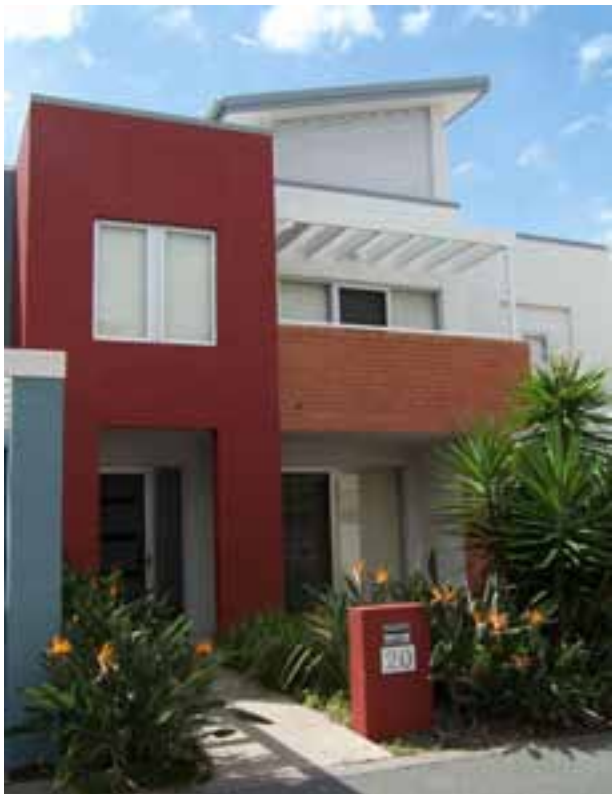
Small front yard, porch, balcony, living spaces and windows fronting the street.
