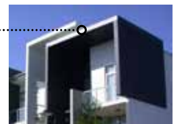
Horizontal Shading device (overhangs) on north facing windows
