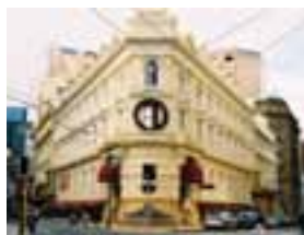
Building at the end of a viewshaft: architectural elements aligned with the centreline of the road
