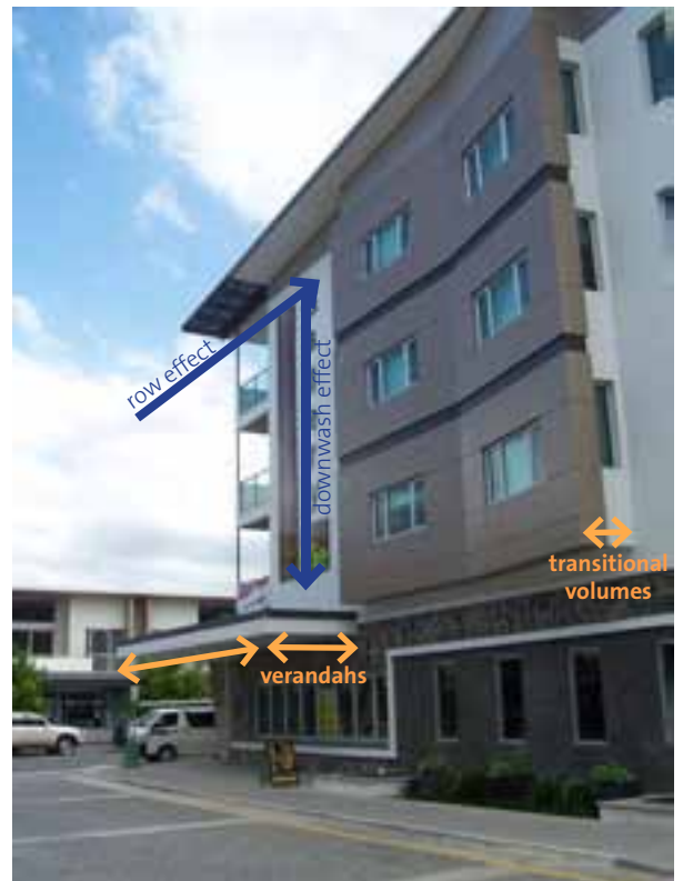
Verandah and transitional volume minimise the adverse effect of increased wind flow
