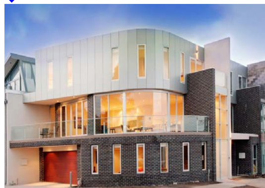
Car parking garage is integrated within medium density residential building and sits back behind a street facade. Garage is a relatively small part of the frontage and is set back from the front wall
