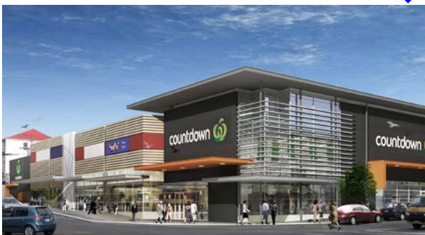
This building has an external facade expressed as a series of forms including a projecting corner form. Various materials and colours emphasise the form variations.
