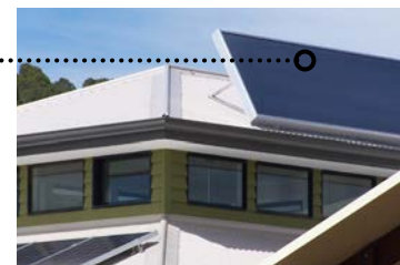
Solar collector devices positioned to maximise sunlight absorption
