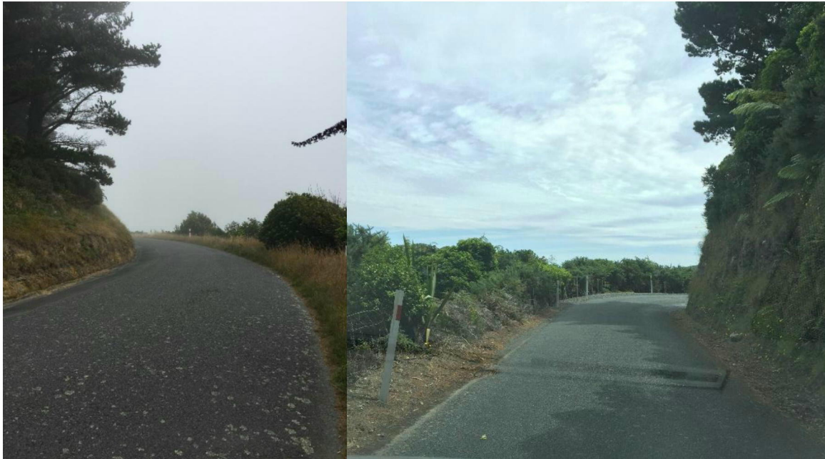
Two representative sections of Normandale Road between numbers 237 and 308
