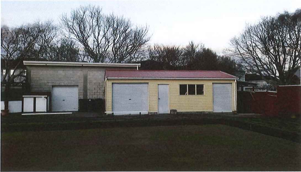
Photograph 3: The implement shed situated in the southwestern corner.
