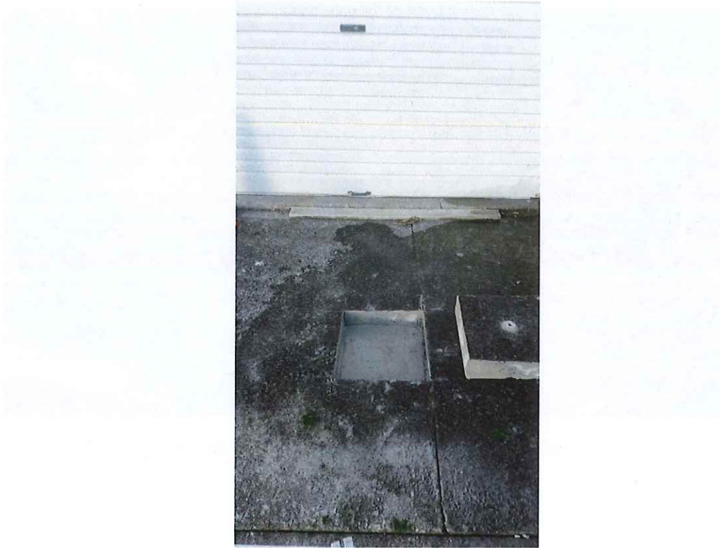
Photograph 5: The historical concrete path still present beneath the present-day path outside the implement shed in the southwestern corner of the site.
