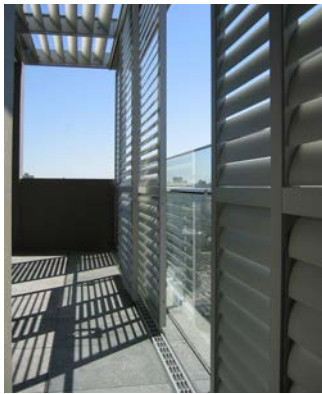
Adjustable screens enable privacy and management of sunlight access/solar gain to residential development (apartment)
