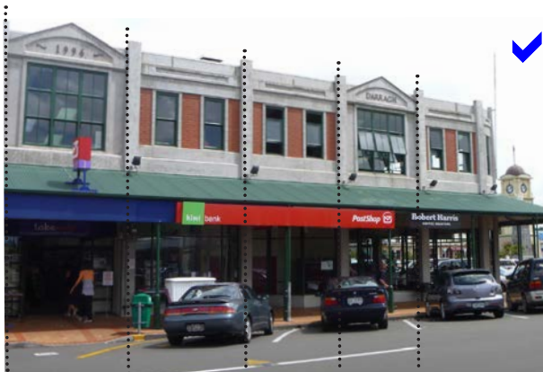
This building is a new block, but has an articulated form of identifiable parts given recessive and projecting elements (dotted lines). It is typical of the character of older buildings and a useful reference for new buildings.
