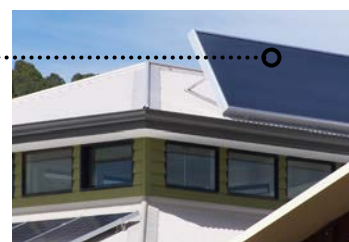
Solar collector devices positioned to maximise sunlight absorption
