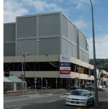
Car parking structure dominates the streetscape, inactive street edge and elongated blank walls
