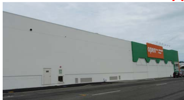
Long blank walls are reflective of utilitarian and internal space requirements. However, these forms can be moderated.
