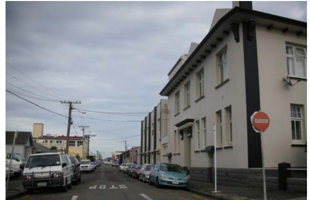
In the area north of Jackson Street the activities are similar in nature to those in Victoria to Sydney Street block. The buildings vary more in height and type and there is a greater mix of set backs and buildings built to the street edge. The street pattern is less regular than the Victoria to Sydney Street blocks.
