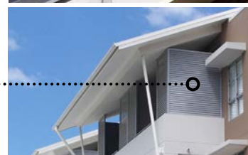
Eaves and moveable vertical shading device (external venetian blind) on east or west facing windows
