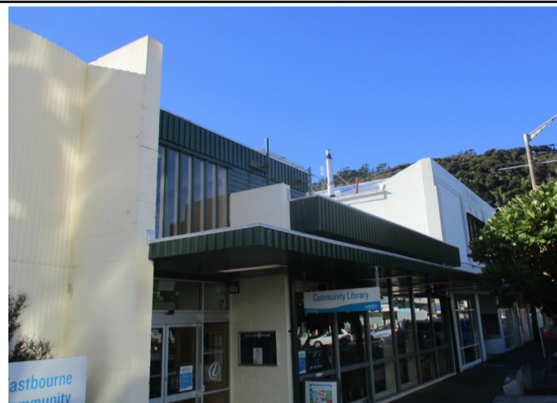
South-West Elevation showing extensive glazing on the ground floor
