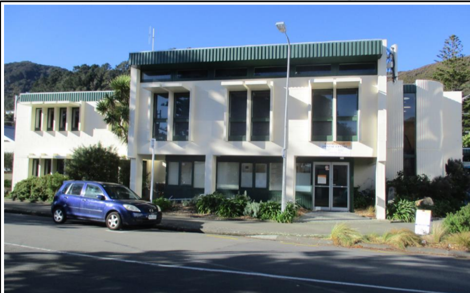
North-West Elevation showing extensive glazing on the ground floor
