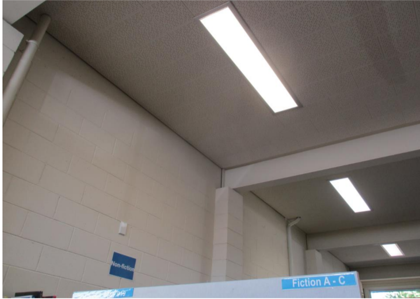
Steel beams span in the transverse direction on the ground floor
