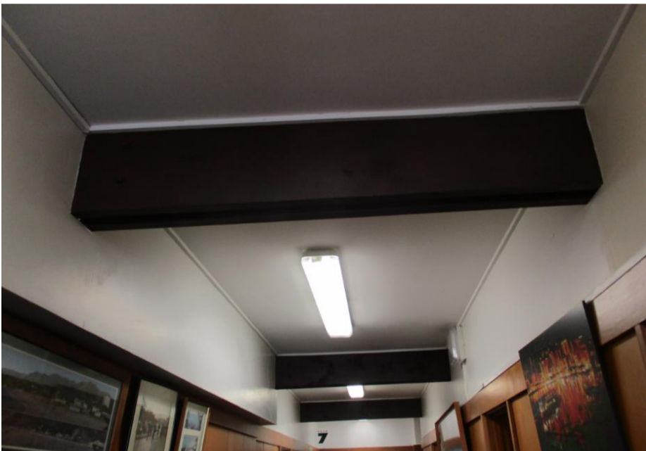
Timber beams span in the transverse direction on the first floor
