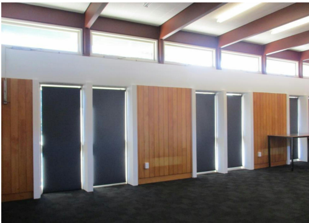
Figure 4 View of the timber-framed construction of the roof structure
