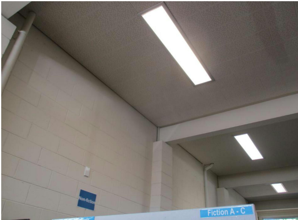
Figure 3 View of the steel beams supporting the first level floor
