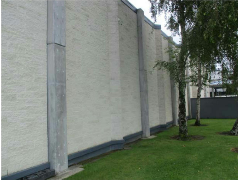
Figure 6 Brick veneer URM wall cladding at south and east elevations
