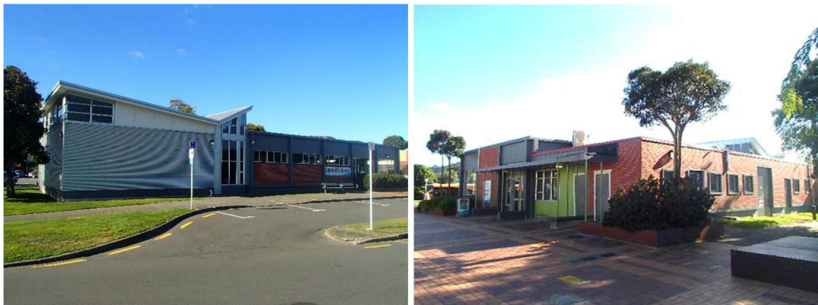
Figure 2: External photographs (NE view and SW view)
