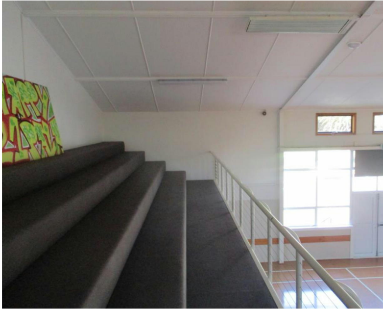
Figure 4 View of braced wall located beside the glazing
