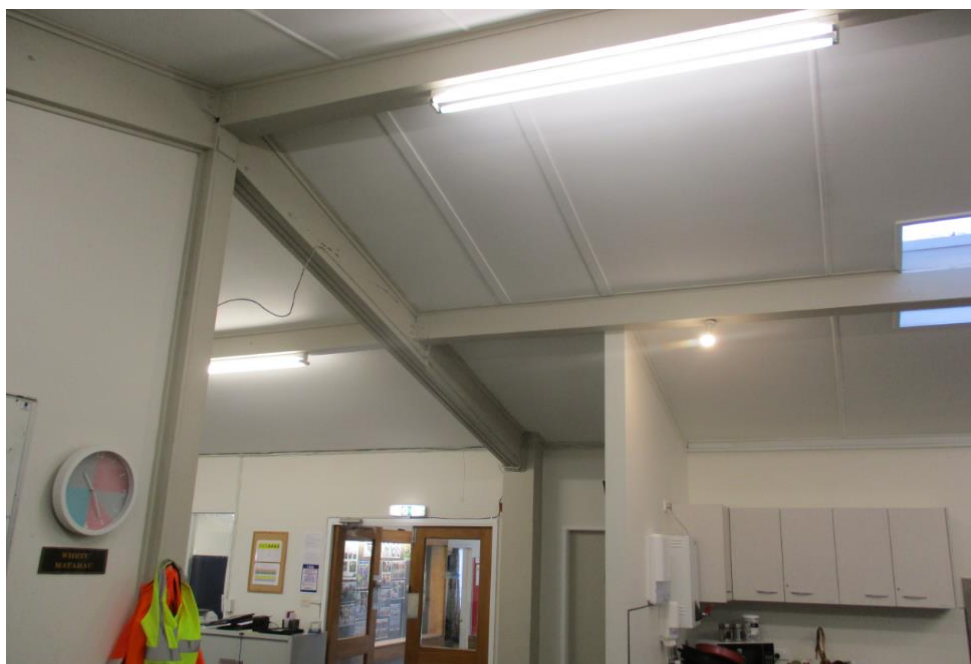
Timber-framed ancillary building
