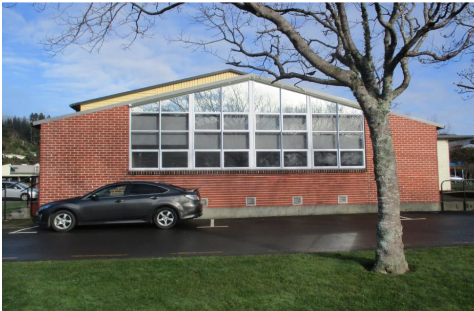
East elevation of the building
