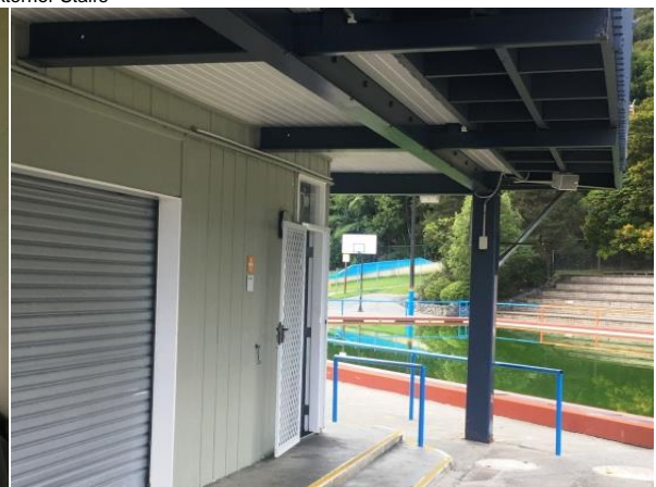
fig 6 - Cantilever Deck & SHS Post
