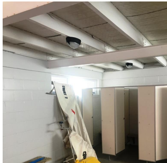
fig 5 - Internal Roof Structure
