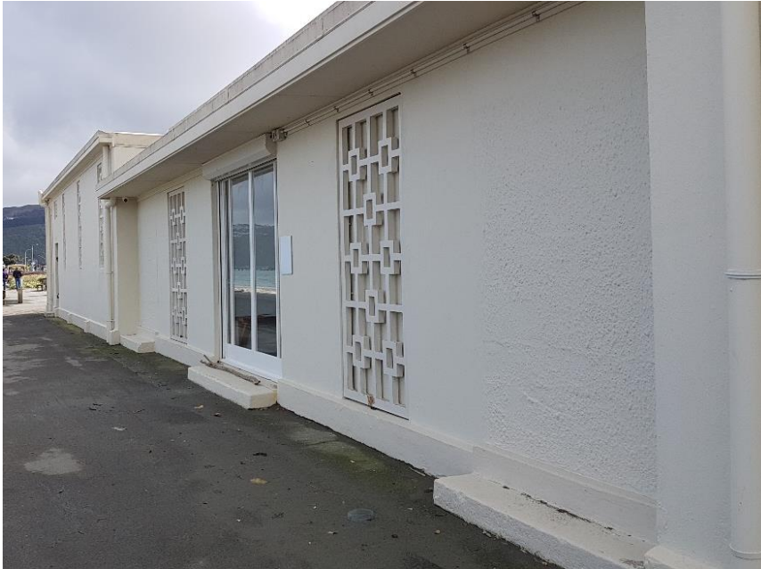
Figure 3: South elevation of Vestibule and Gallery Wing.
