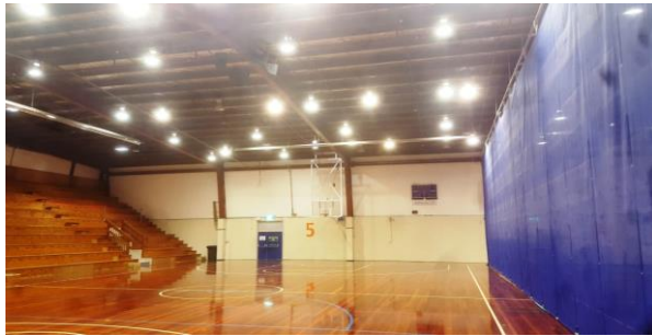
fig 1a.1 inside gymnasium (portal frames & tiered seating)
