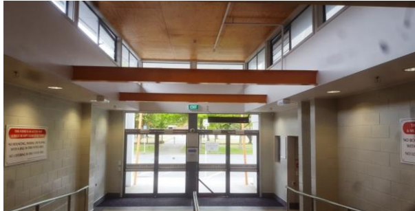
fig 1a.2 inside the north-west entry (2002 addition)
