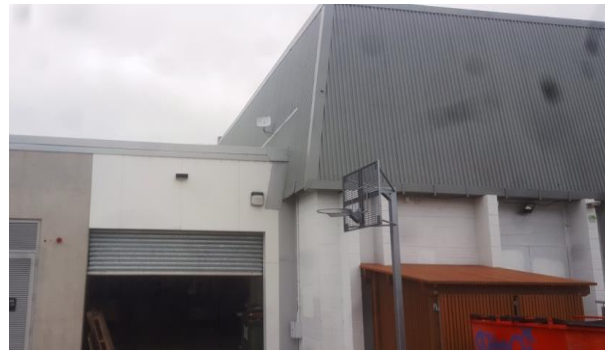
fig 1a.4 outside the south-east wall (seismic gap to the 2013 building to the south)
