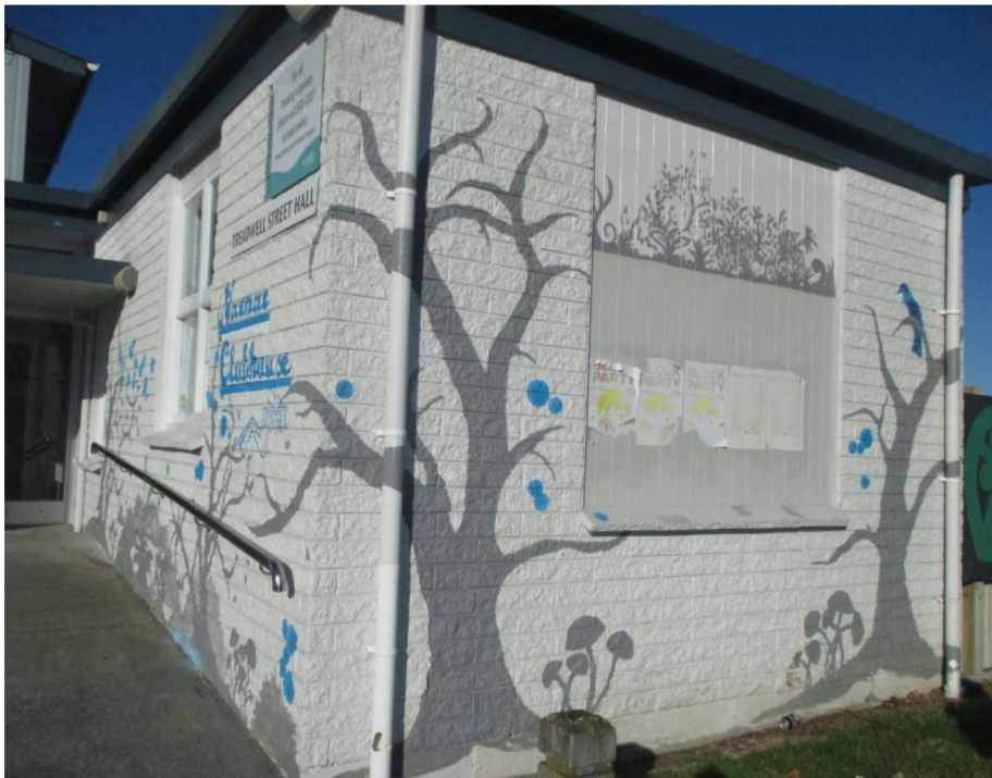
Figure 5 Brick veneer cladding to the north end of the building
