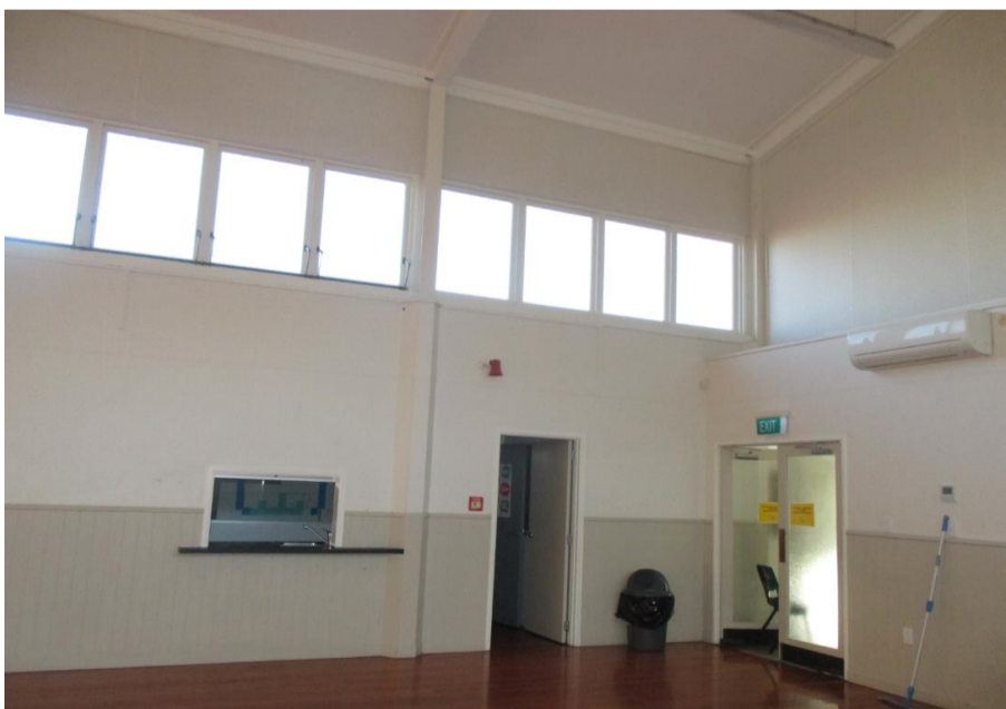
North and west timber walls
