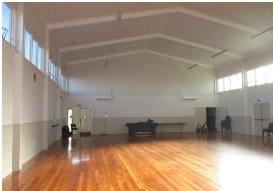
Steel portal frames in the building
