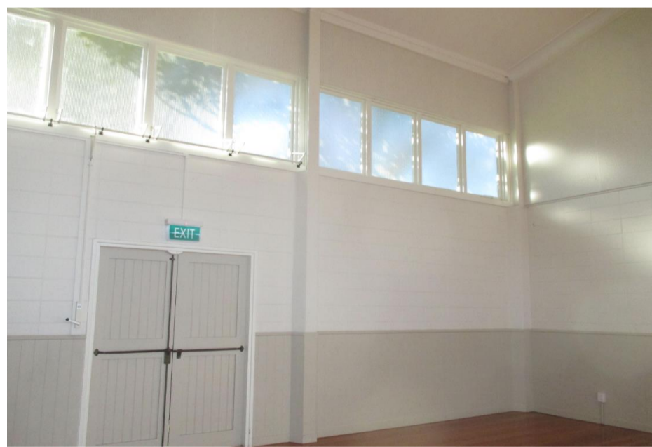
South and east masonry walls
