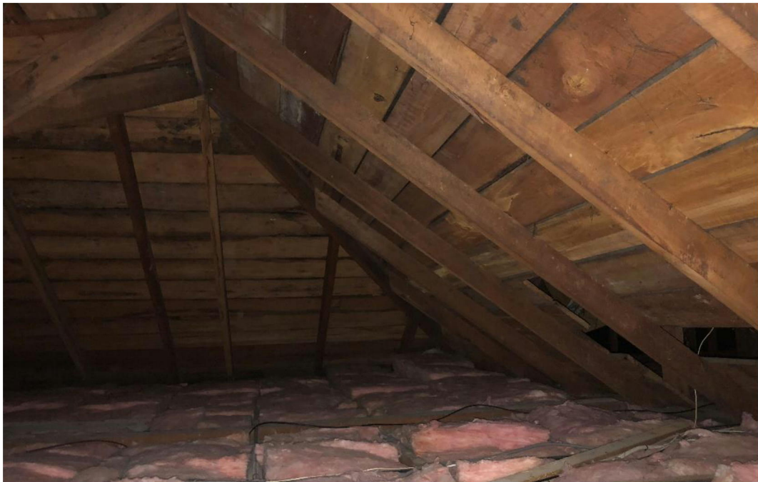
Figure 4 Sarking and ridges of roof
