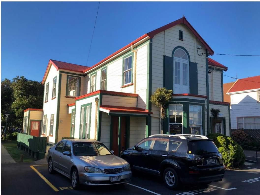
Figure 3: Front view of Petone Community House
