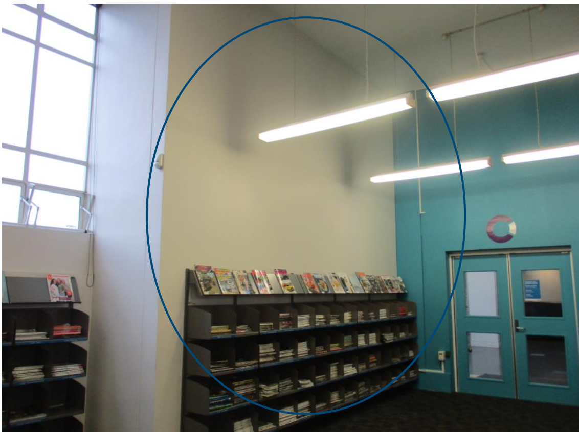
Example of RC shear wall
