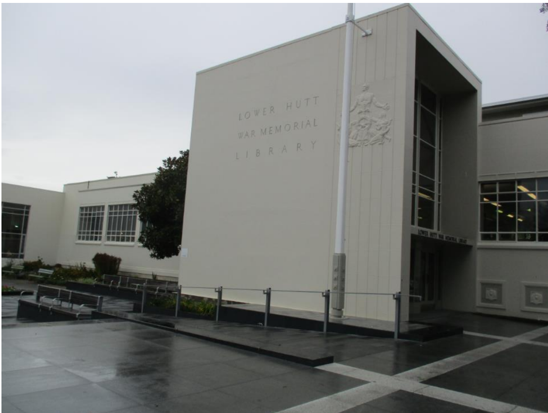
North elevation of the building
