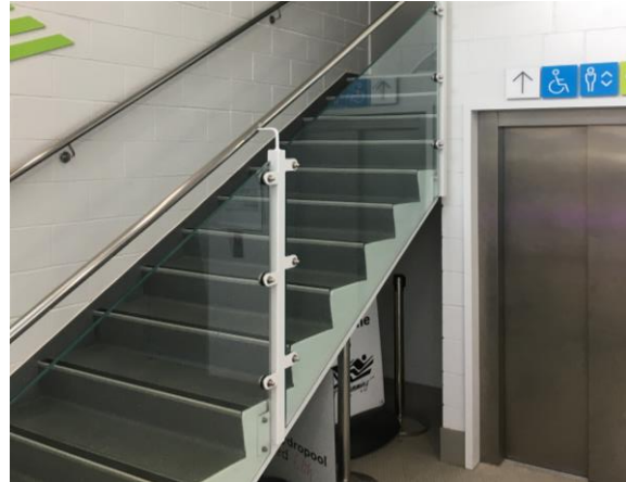
fig 2 - Pre-cast stairs and reinforced concrete lift core.
