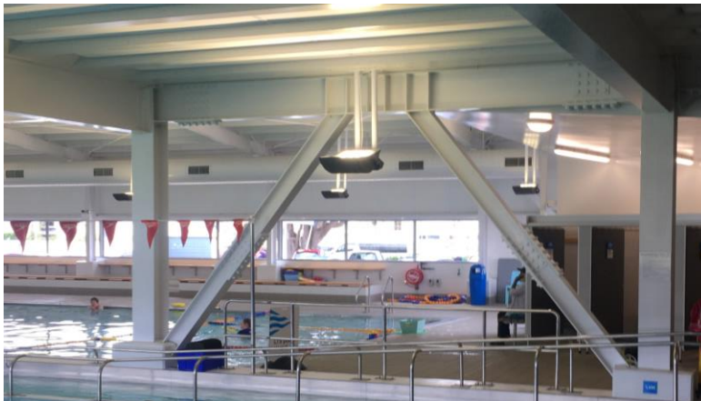
fig 3 - Eccentrically braced frame and interspan floor above.
