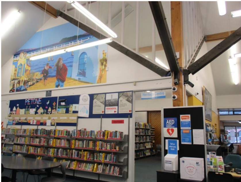
Figure 4 Twin struts and ring beams
