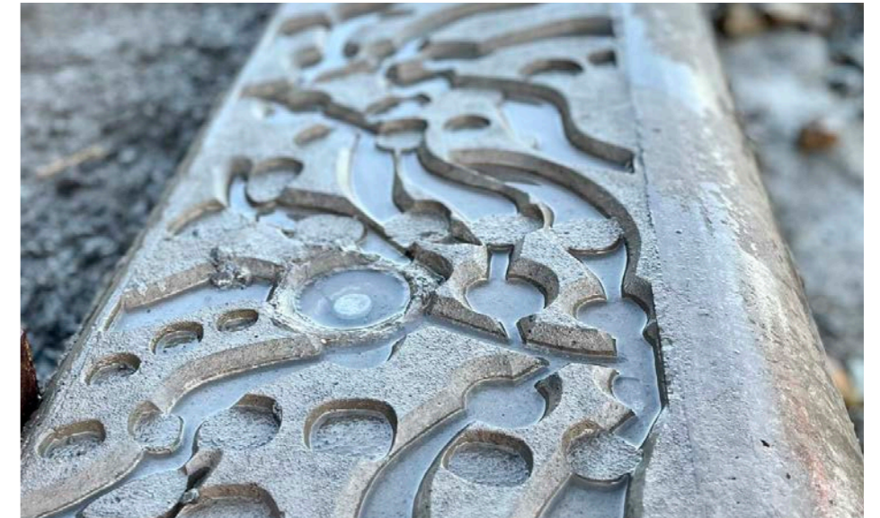
Figure 1.13 Texture applied to the curved seawalls
