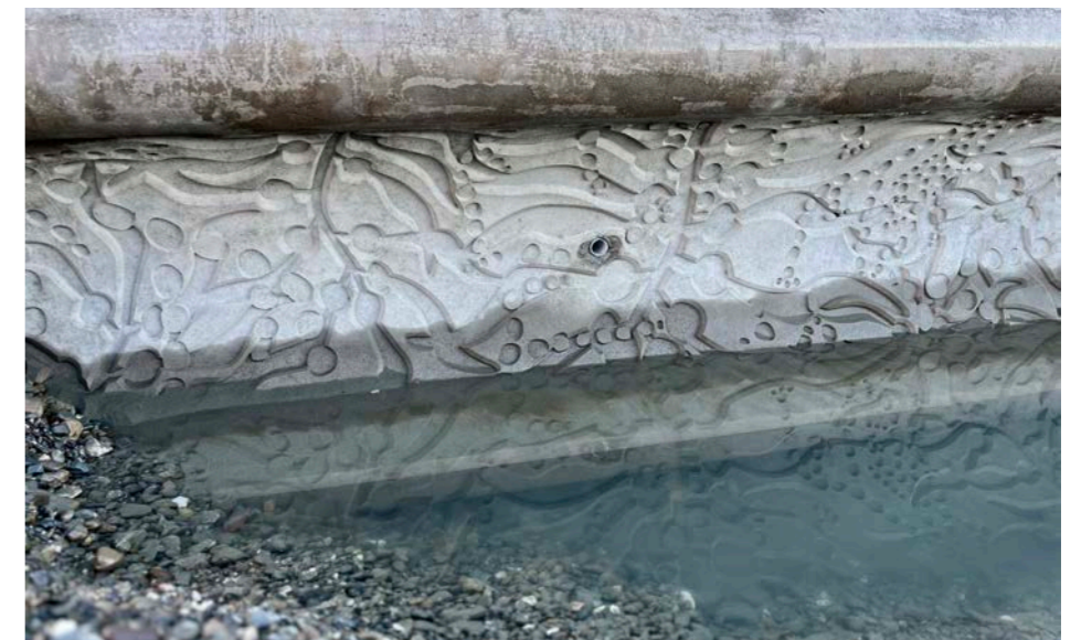
Figure 1.14 Texture applied to the curved seawalls
