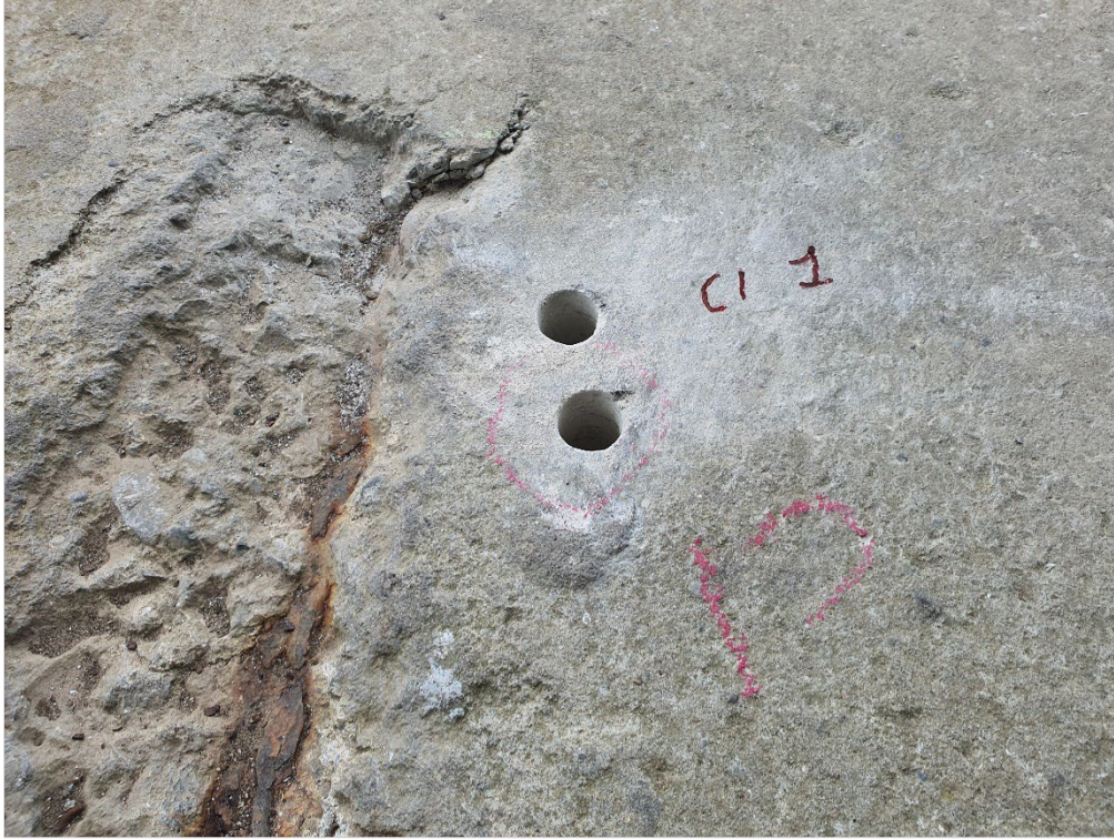
Figure 72: Chloride testing location Cl.1
