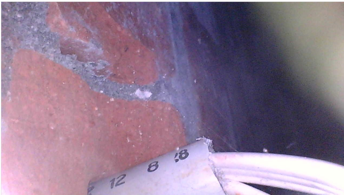
Figure 82: Wall between column 2&8
