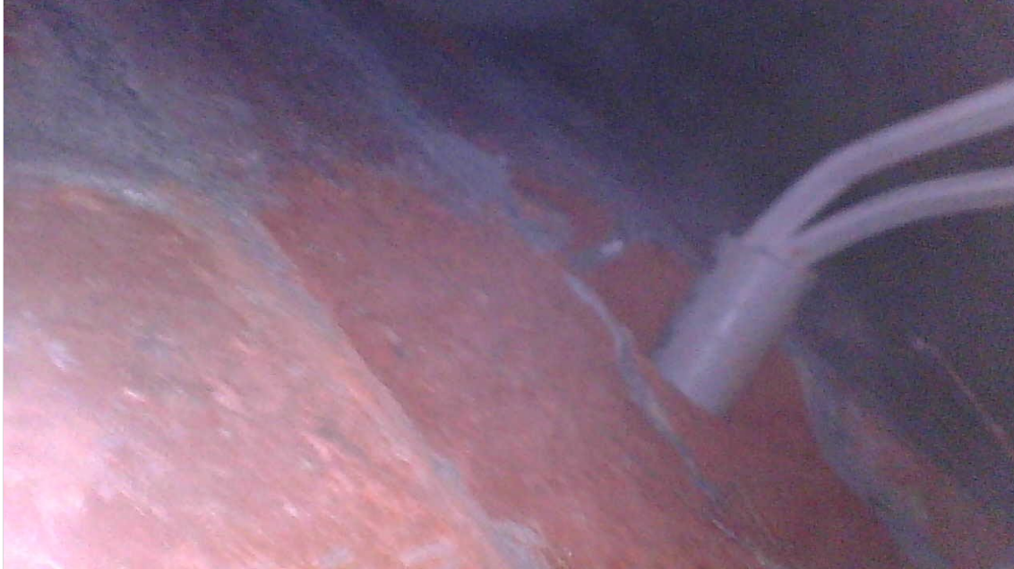
Figure 81: Wall between column 2&8
