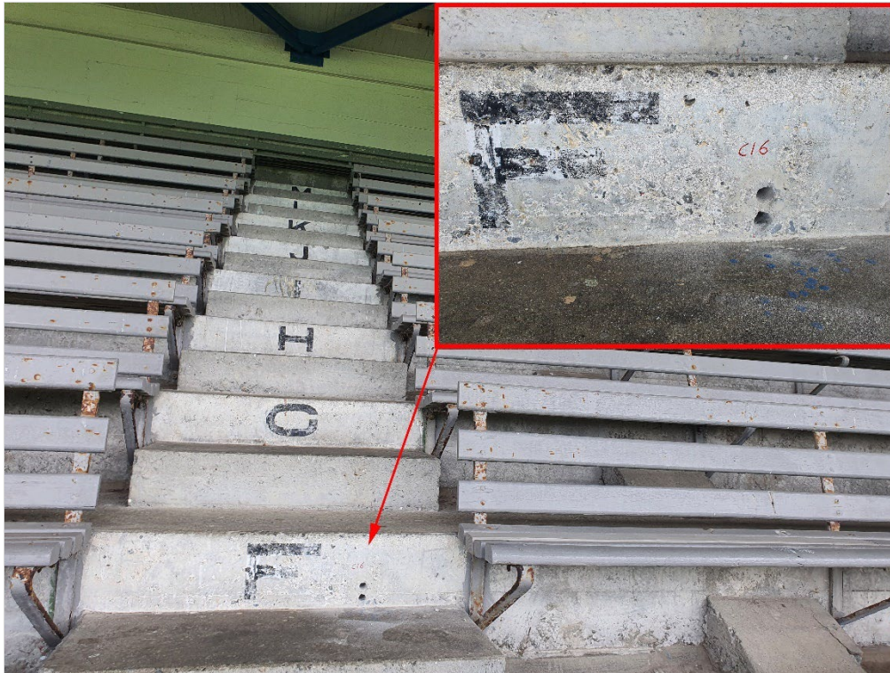
Figure 77: Chloride testing location Cl.6
