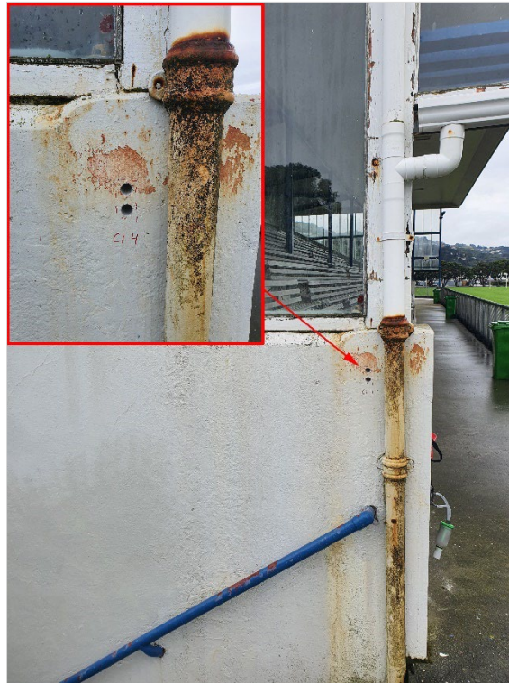
Figure 75: Chloride testing location Cl.4
