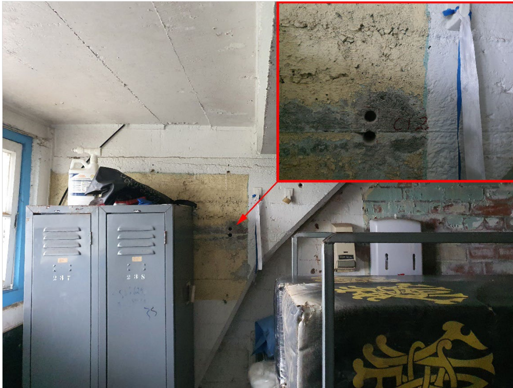
Figure 73: Chloride testing location CI.2
