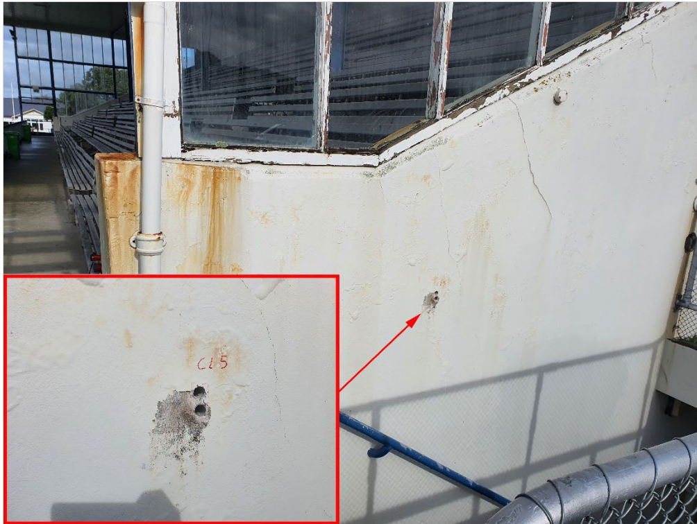
Figure 76: Chloride testing location CI.5
