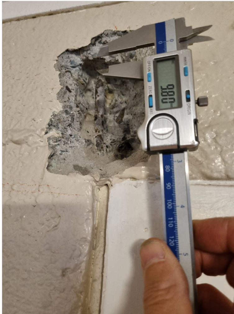
Figure 85: Lintel - grid D breakout
