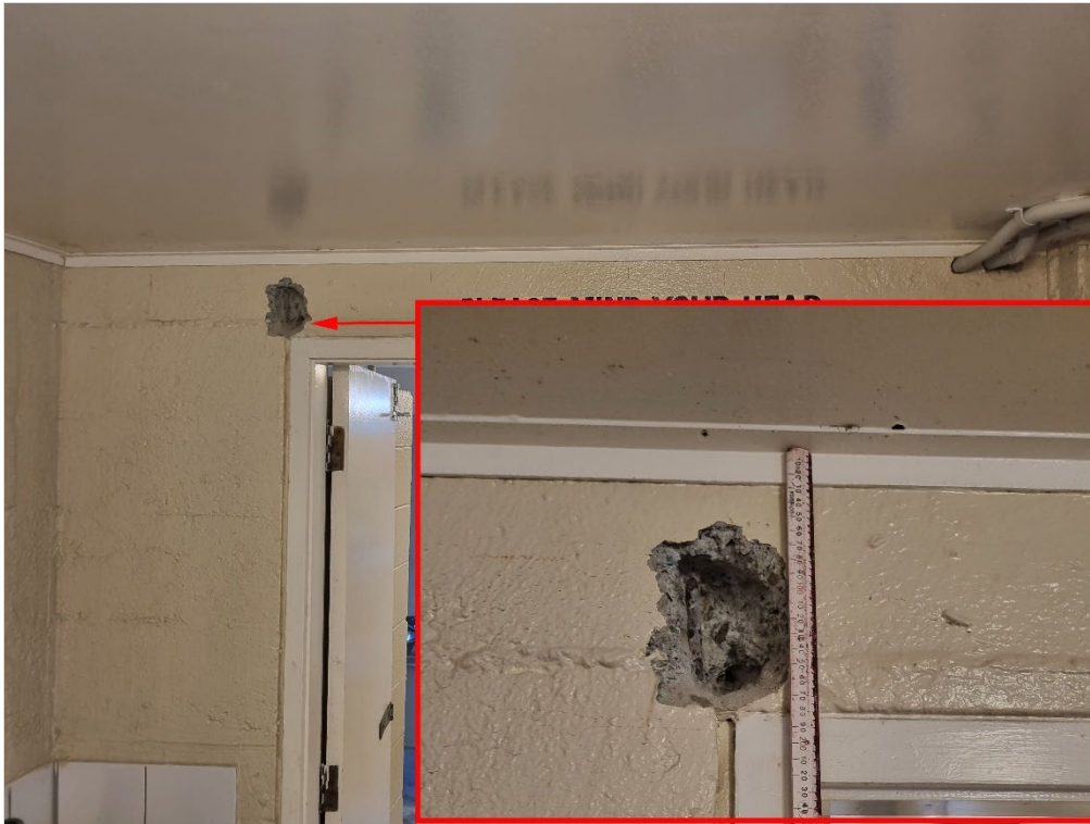
Figure 84: Lintel – grid D
