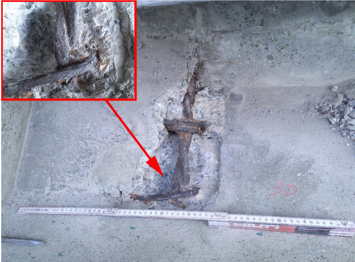
Figure 48 Location 3d - Breakout
