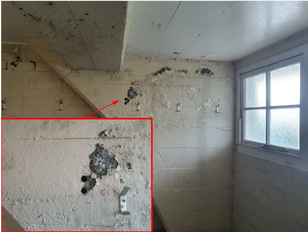
Figure 74: Chloride testing location CI.3
