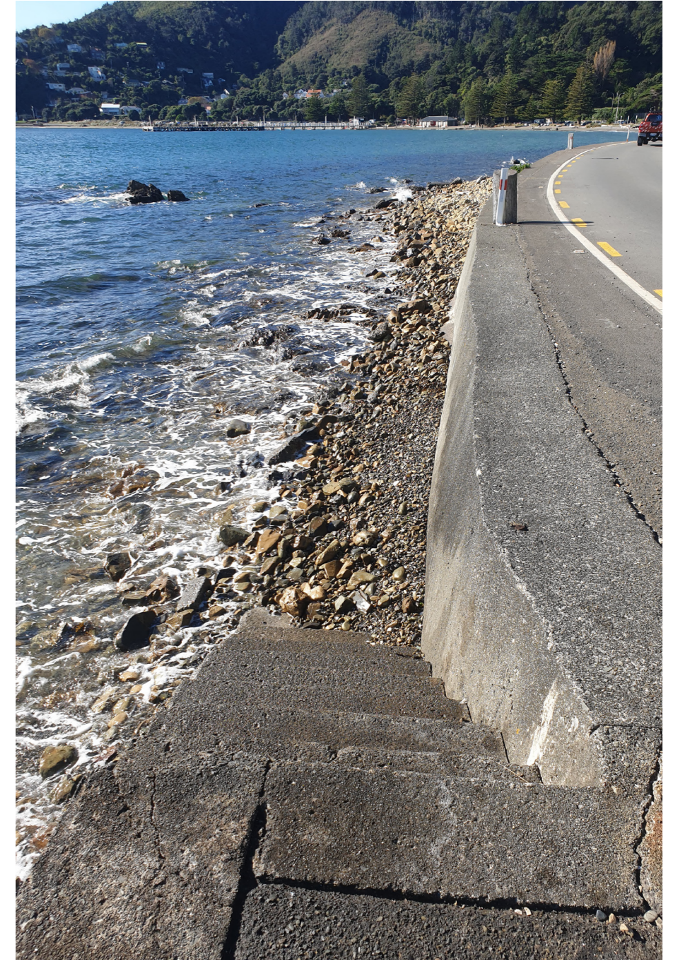
Figure 1.8 Existing stairs down to beach area at Mā-Koromiko
