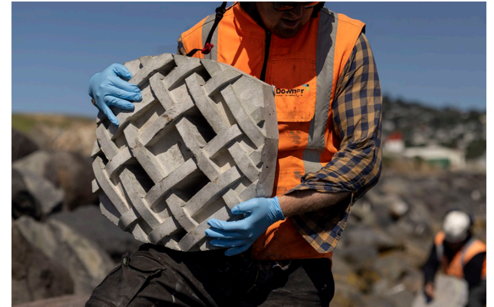
Figure 1.14 Ecological tiles, to be added at discrete locations along vertical surfaces at steps and landings within the intertidal zone.
