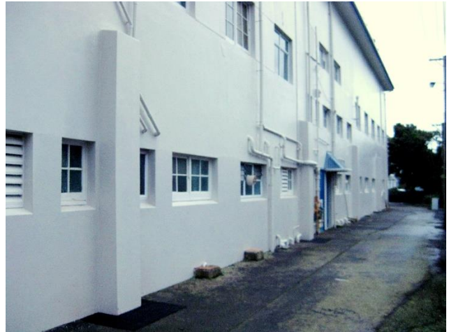
Figure 3 - Exterior North-West Corner
