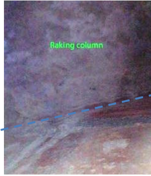
Figure 21 - Height of the Unreinforced Masonry (URM) Infill Wall - Btn Col 4 & 10 at Ground Floor.
