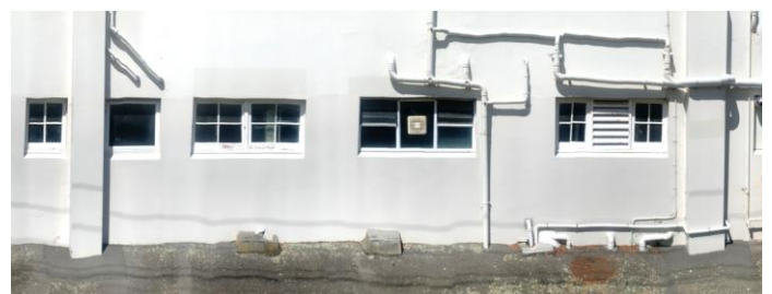
Figure 29 - Photograph of the back wall between columns 16 and 17.
