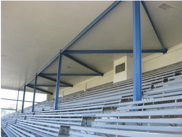
Figure 2 - Grandstand Seating with 1979 Roof Bracing Above
