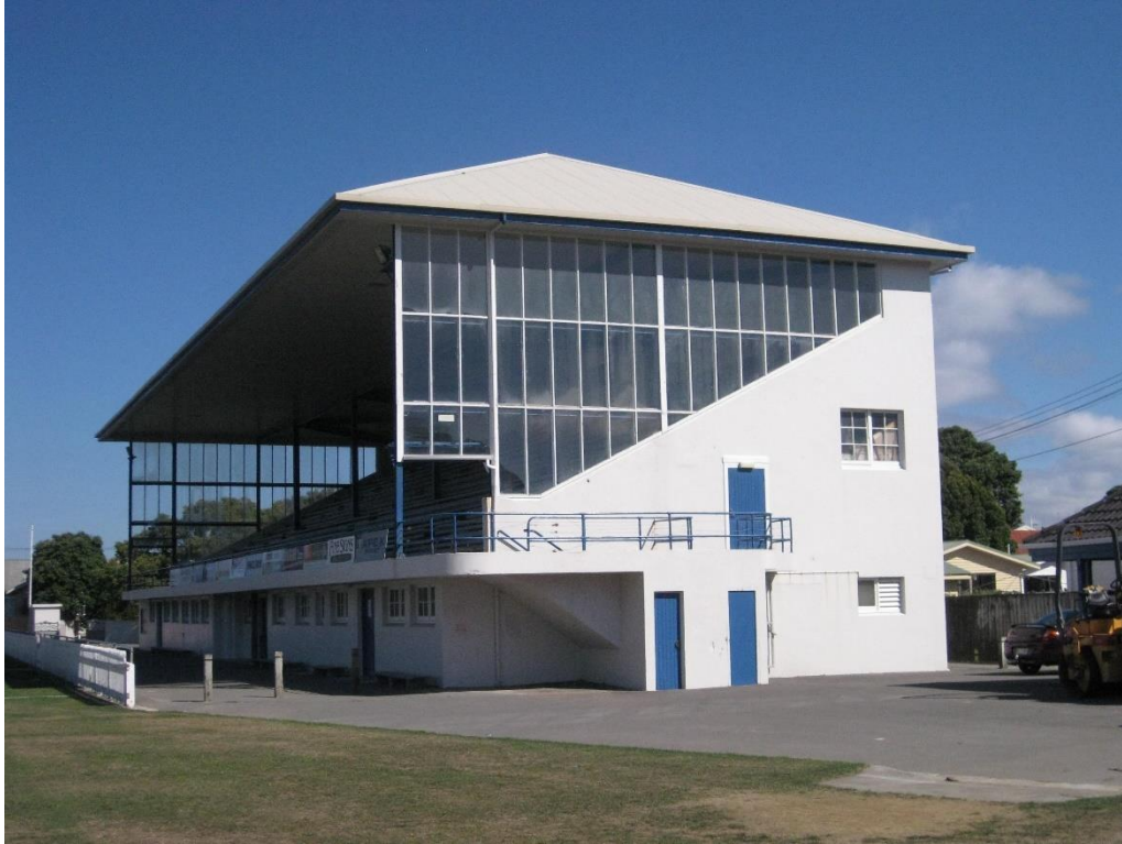
Figure 1 – Photograph of the building from the east.
