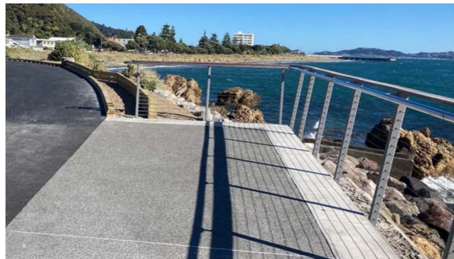
Figure 1.15 Completed balustrade at southern end of Mā-koromiko.
