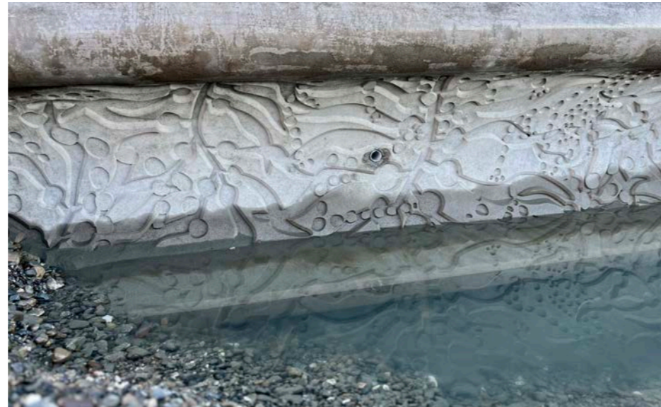
Figure 1.17 Texture applied to the curved seawalls
