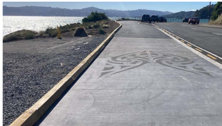
Figure 1.16 Completed timber kickstand.
