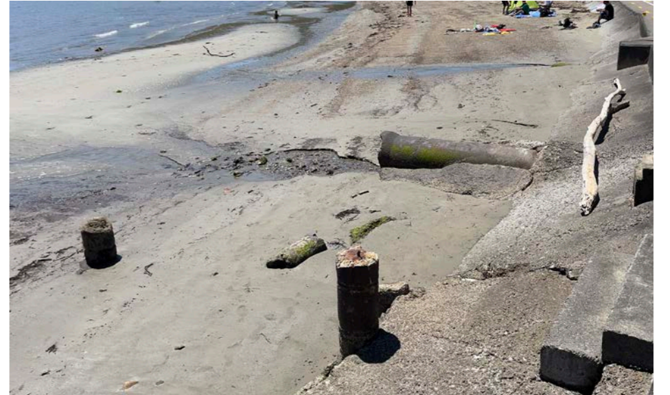
Figure 1.6 Existing stream and culvert in Whiorau Bay
