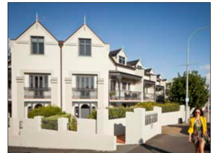
High quality terraced housing envisaged along Cornwall Street creating an attractive interface with the centre
