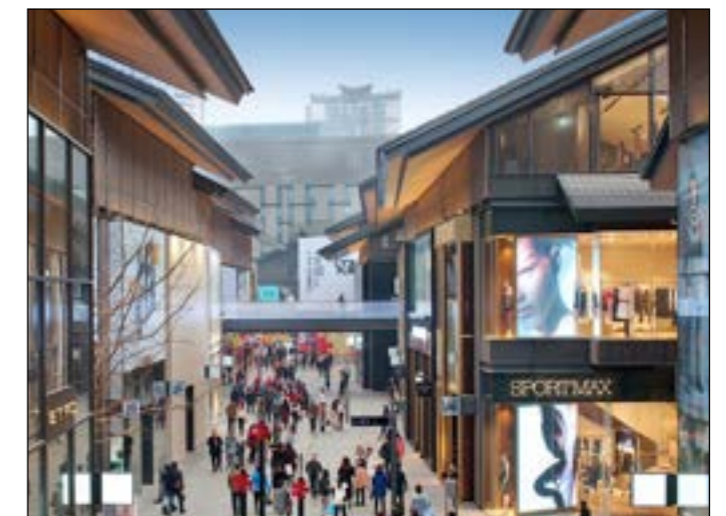
Sino-Ocean Taikoo Li Chengdu (Oval Partnership). New east-west laneways will connect the centre to Riverlink
