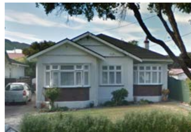
14 St Albans Grove (not DP Listed)
