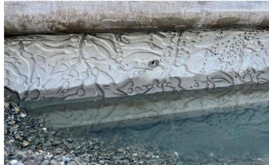
Figure 1.24 Photo of ecological enhancement texture applied to curved seawalls vertical faces.
