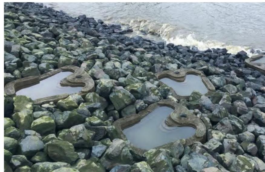
Figure 1.25 Tide pools installed in rock revetment. Ref SHRP
