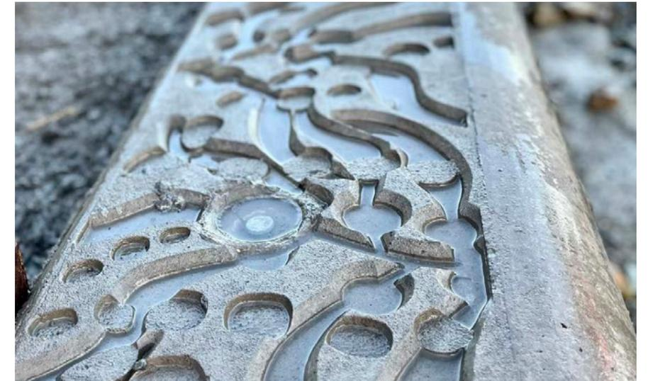
Figure 1.23 Photo of ecological enhancement texture applied to concrete seawalls horizontal faces.
