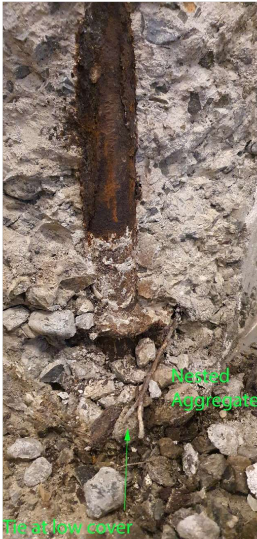
Figure 43: Column Grid B-Y - Breakout
