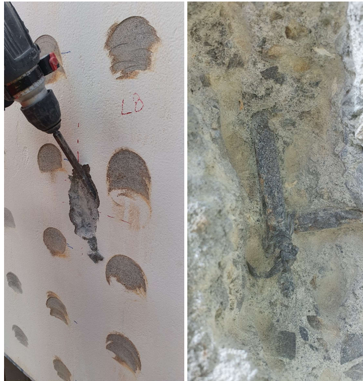
Figure 35: West Wall – Grid A-B - Breakout L8
