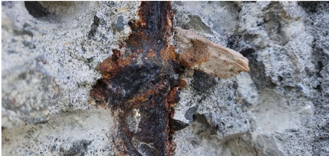
Figure 19: West Wall – Grid E-F - Breakout L1
