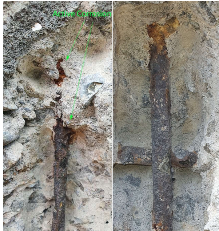
Figure 34: West Wall – Grid A-B - Breakout L7
