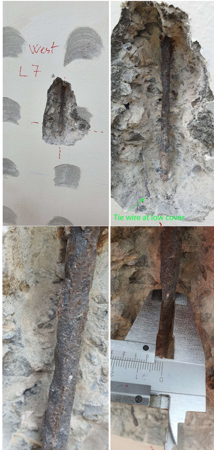
Figure 33: West Wall – Grid A-B - Breakout L7
