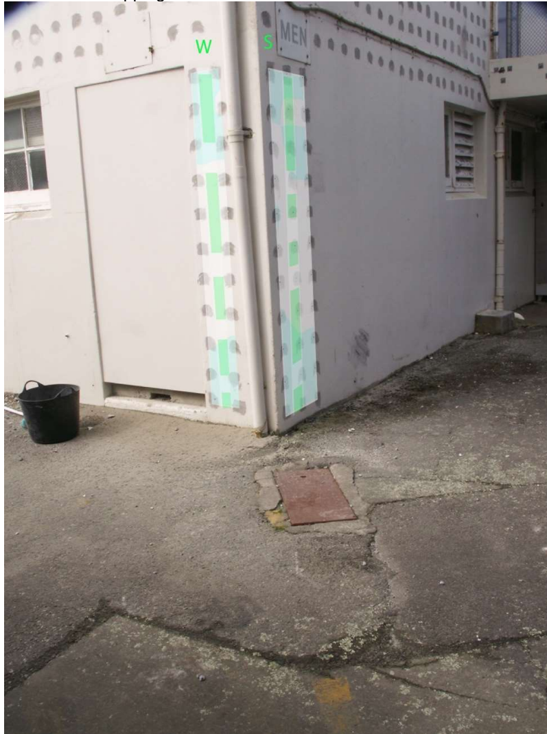
Figure 39: Column A-Z - Half-Cell - Cover Map
