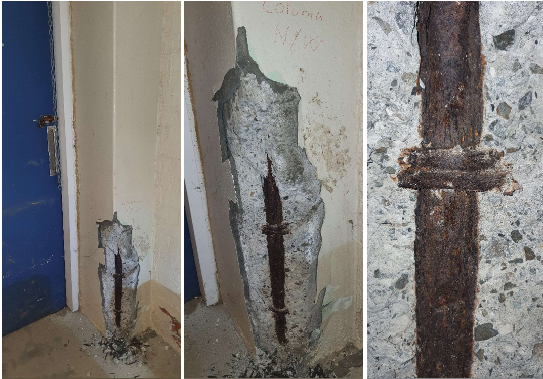
Figure 60: Column Grid F-Z - Breakout Location
