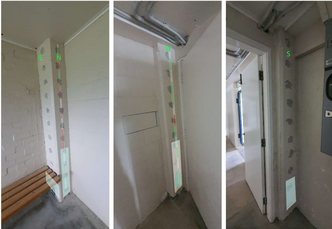
Figure 52: Column D-Y - Half-Cell - Cover Map
