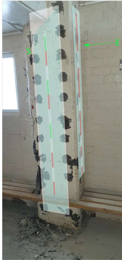
Figure 57: Column Grid F-Y - Half-Cell - Cover Map
