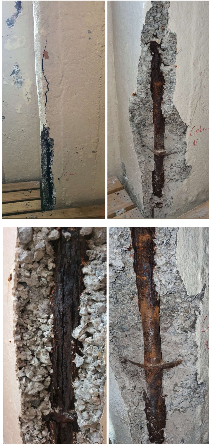
Figure 58: Column Grid F-Y - Breakout Location
