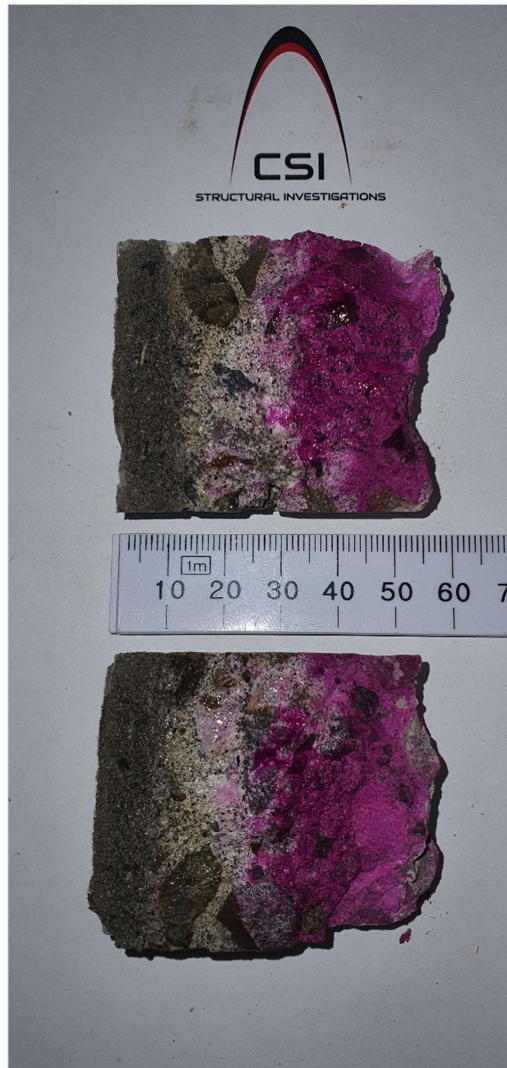
Figure 18: West Wall Grid E-F - Carbonation Testing
