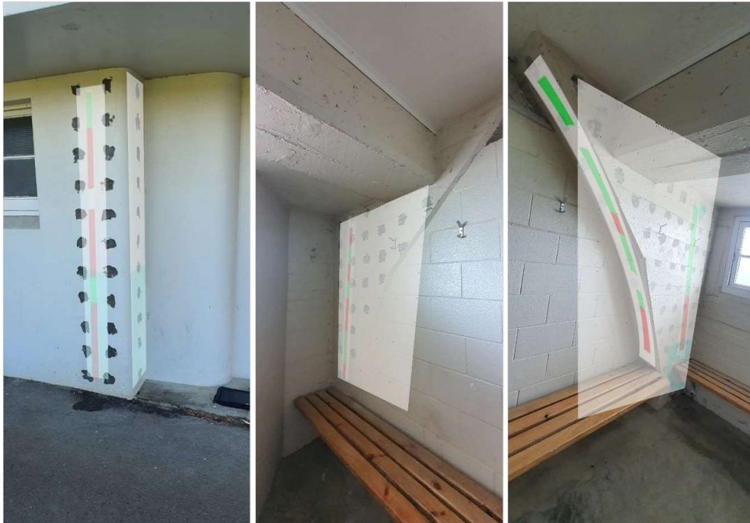
Figure 49: Column Grid C-X - Half-Cell - Cover Map
