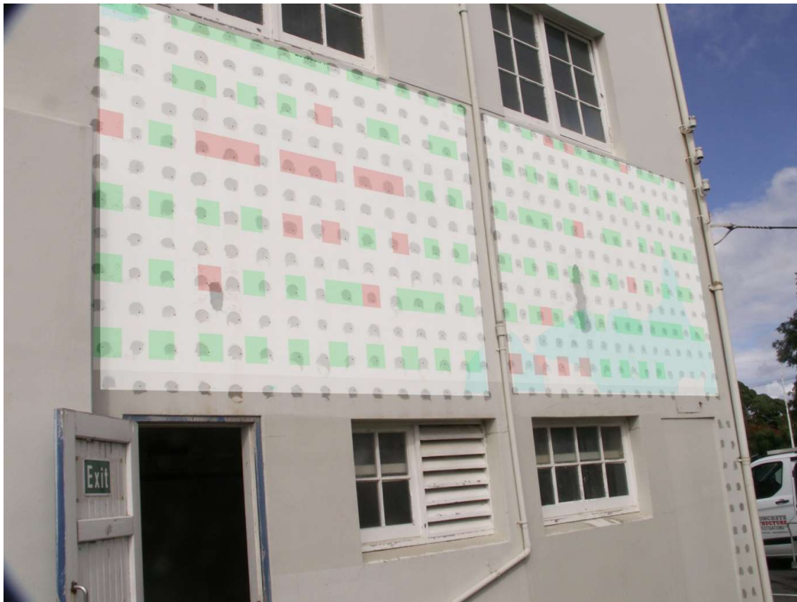
Figure 30: West Wall Grid A-B - Half-Cell - Cover Map
