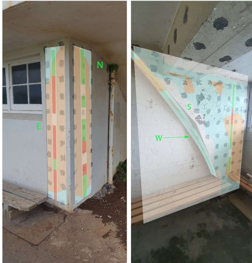
Figure 56: Column Grid F-X - Half-Cell - Cover Map
