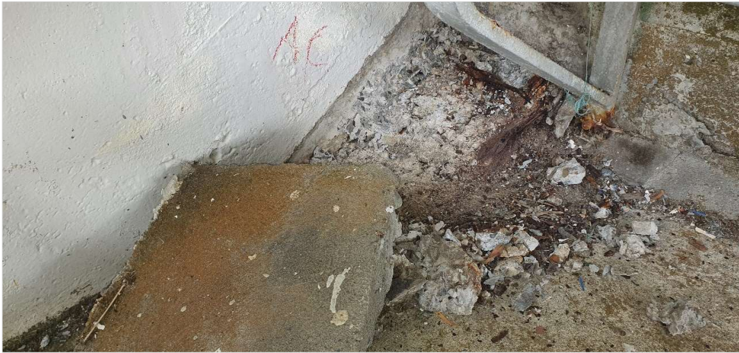
Figure 73: Raking Beam AC - Condition
