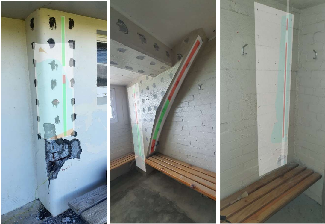
Figure 51: Column D-X - Half-Cell - Cover Map
