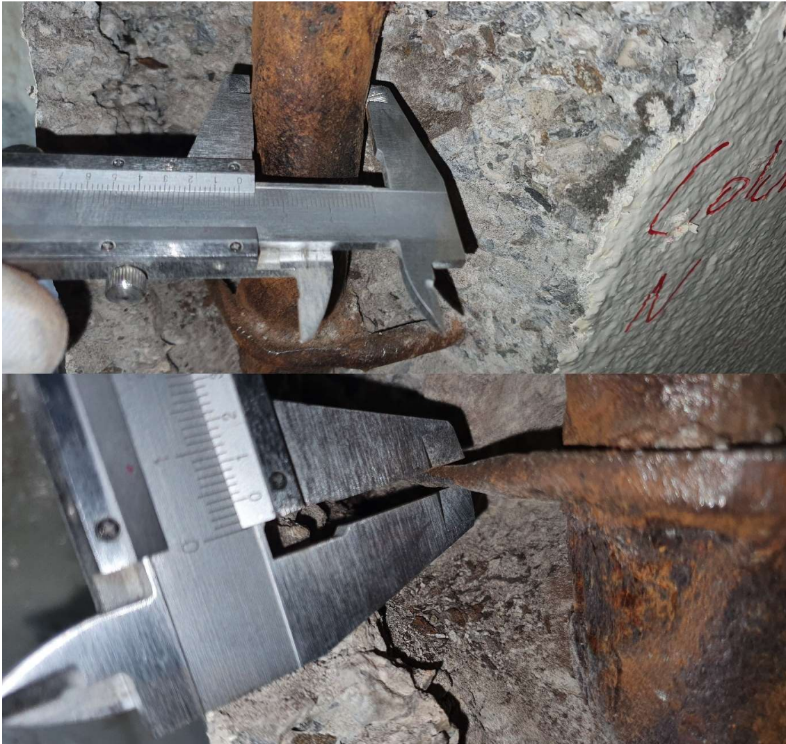
Figure 59: Column Grid F-Y - Breakout Location
