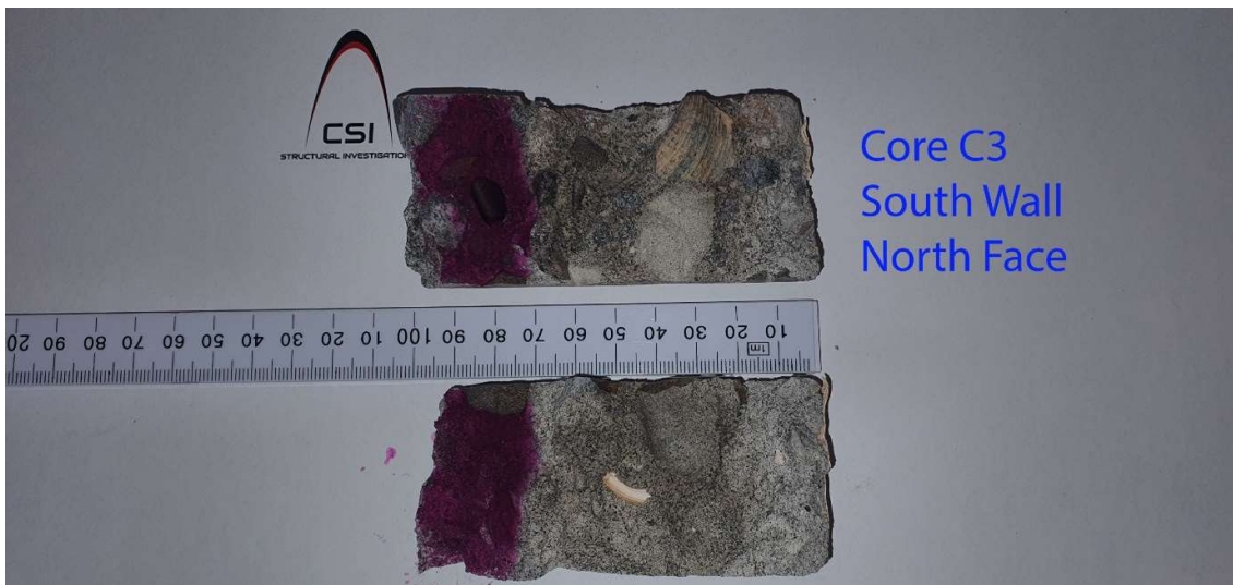
Figure 6: South Wall / North Face - Carbonation Testing
