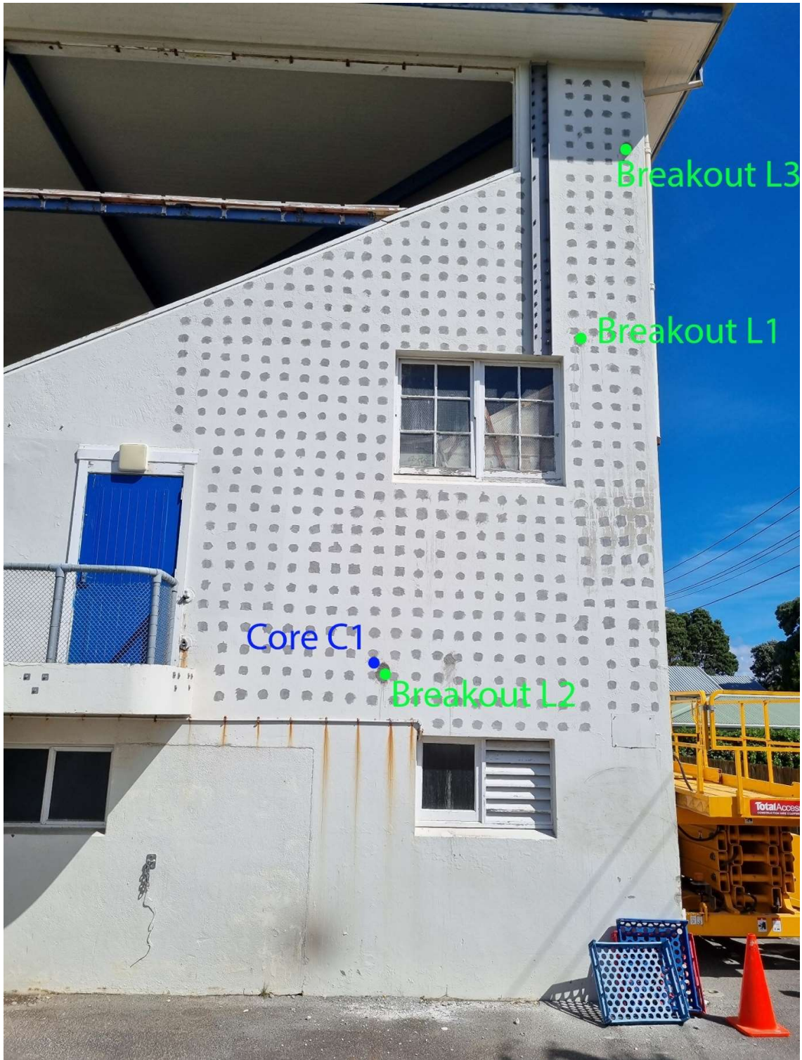
Figure 12: North Wall - Core and Breakout Locations
