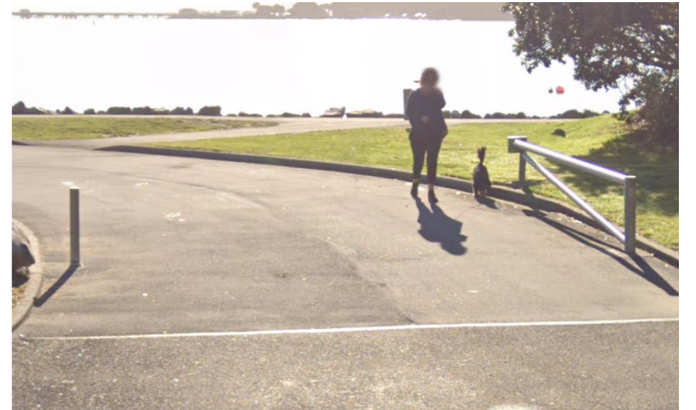
Figure 1.10 Existing vehicle barrier to be retrofitted with mesh screen extending to ground level
